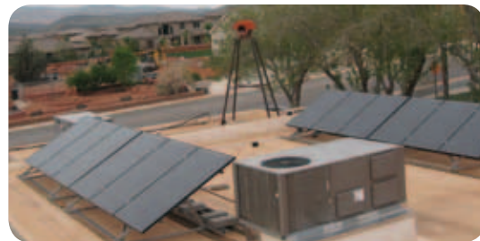
Solar panels on the Ivins community fire station
