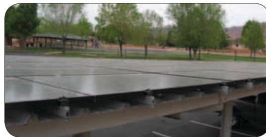
Solar panels on the parking structure next to Ivins City Hall
