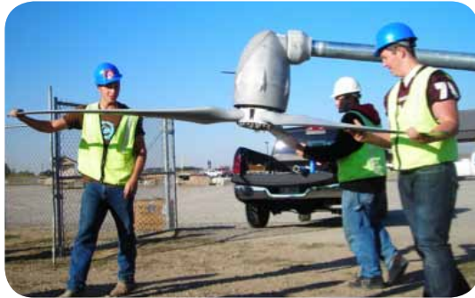
Installation of wind turbines for Rigby High and Midway Middle School in Idaho
