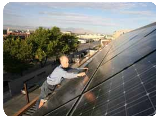
Solar array installed at Salt Palace in 2006
