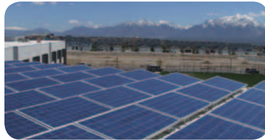
Blue Sky funds helped bring this 10.1-kilowatt solar array online at Early Light Academy in South Jordan, Utah.
