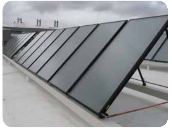
Solar water heating panels at the J.L. Sorenson Recreation Center
