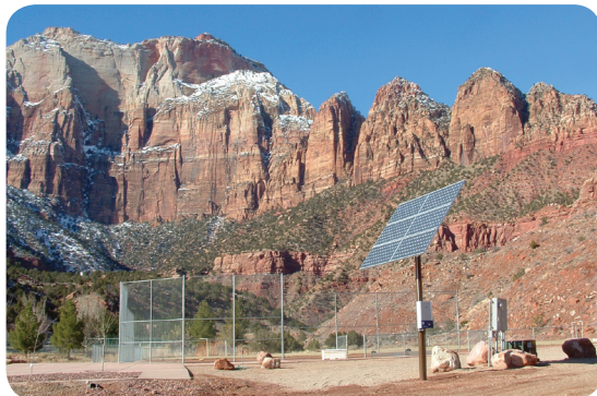
A solar panel powers a baseball field in Springdale, Utah.
