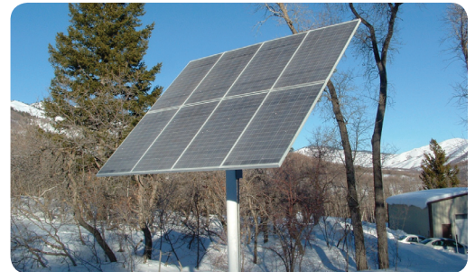
Solar panel at The Swanson Environmental Center in Eden, Utah
