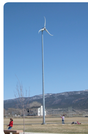
Three Peaks Elementary students made a real difference with a wind turbine installed on the school grounds.
