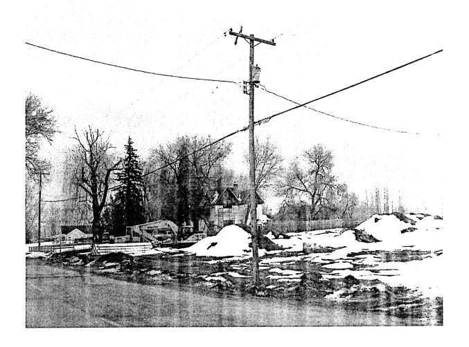
Pole 11206002.0 279904 to 260902 on 2700 W & 1800 S, New cable being placed without resolving existing road clearance violation. No make ready requested, secondary service needs to be raise so attachment can be raised for roadway clearance and maintain 40" clearance at pole. CATV also needs to place anchor and down-guy.
