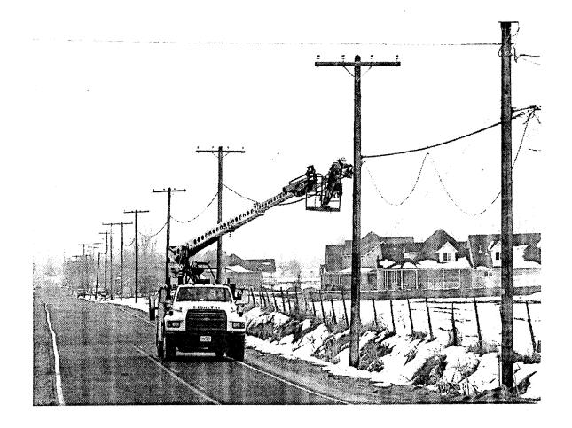
ComCast has placed strand and fiber in violation of NESC clearances and has created a very unsafe condition. A moderate wind will place ComCast in contact with PacifiCorp open wire secondary and energize the ComCast messenger. This eminent hazard will be corrected by PacifiCorp at ComCast expense.
