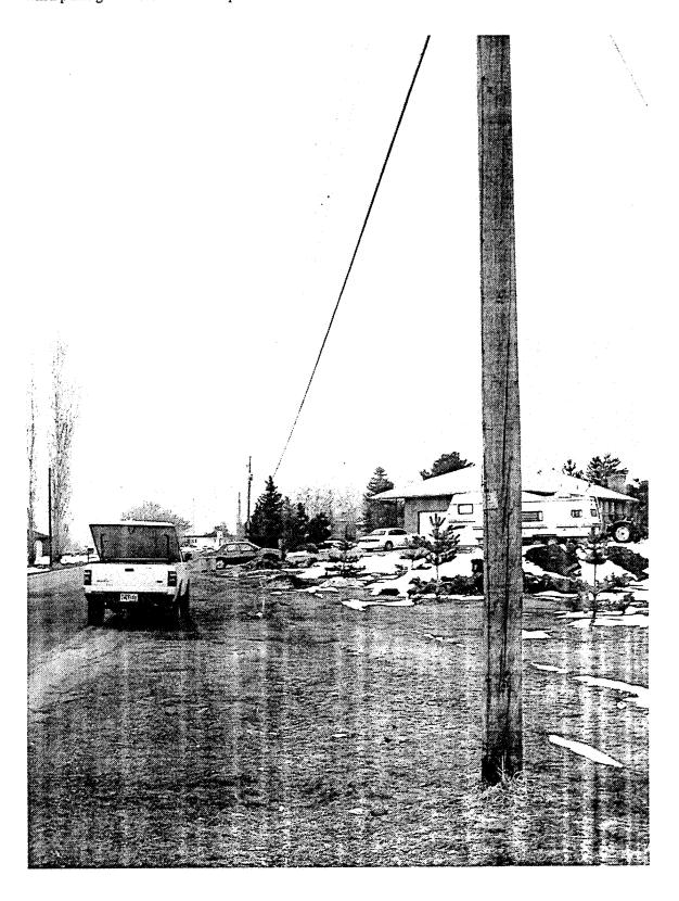
Pole 11206002.0 260500 to 260502, inadequate ground clearance., no make ready prior to placing additional cable.
