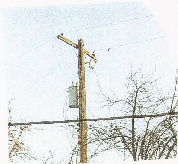
Photo 23 1 failing insulator 2018 E. Lambourn Ave
