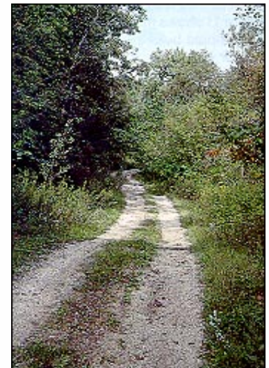
Figure 4. A drainage dip is effective in controlling water on the road and does not significantly slow the speed of vehicles.
