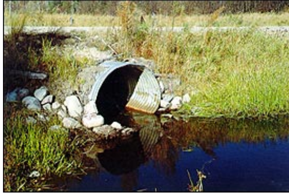
Figure 4. Culverts not installed at the same level as the stream cause water to back up.
