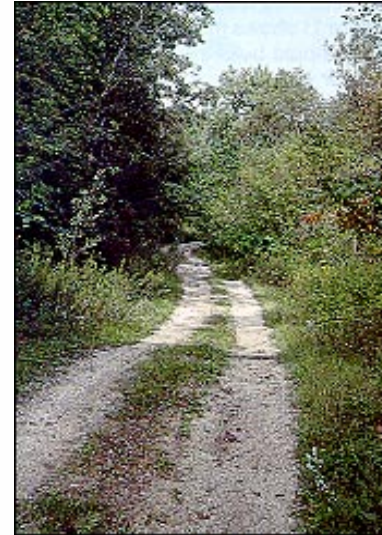
Figure 3. A drainage or rolling dip is effective in controlling water on the road and does not significantly slow the speed of vehicles. (See TA 502)
