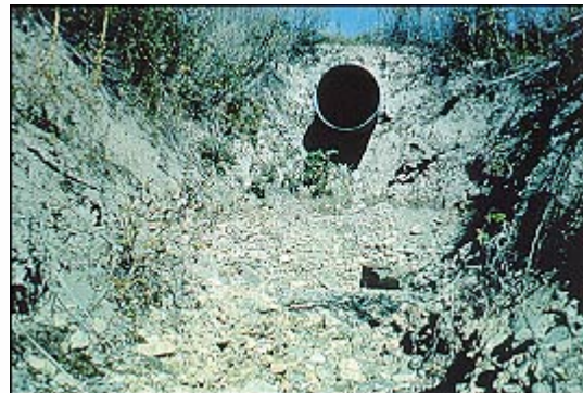
A culvert not installed at the existing stream gradient can degrade the stream channel.
