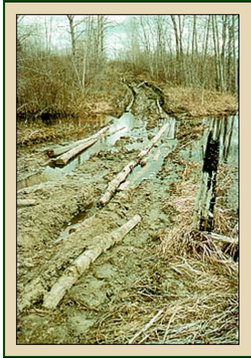
Figure 7. Poor road construction practices in wetland areas can cause problems during construction.
