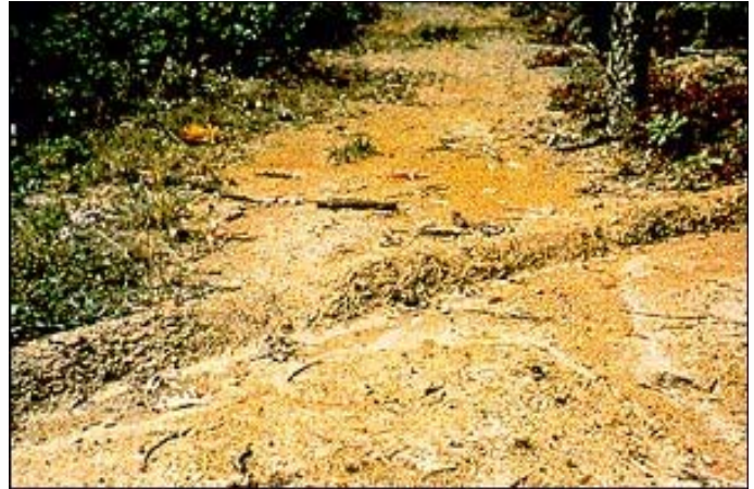
Figure 1: A water bar effectively intercepts surface water and diverts it from the road
