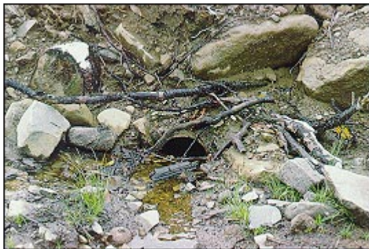
Figure 5. Undersized culverts can become plugged with sediment.
