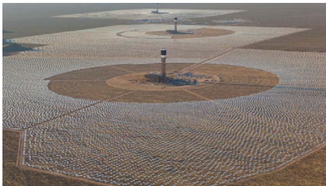
Figure 30. Concentrating solar power plant in the Mojave Desert
