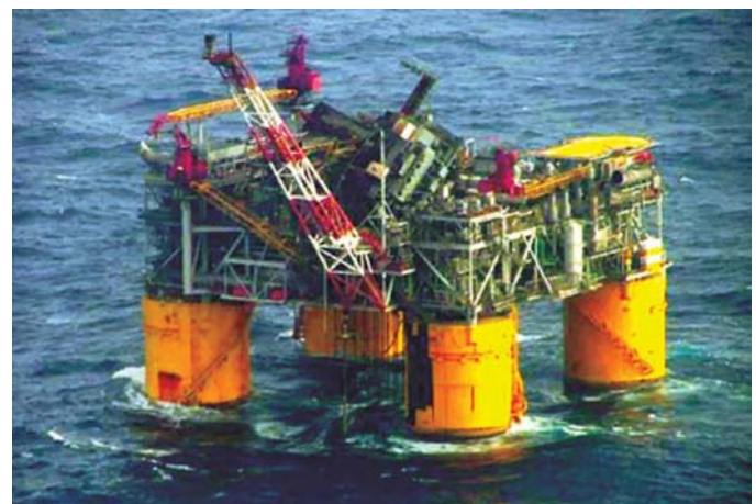
Figure 20. Damaged offshore platform after Hurricane Katrina
