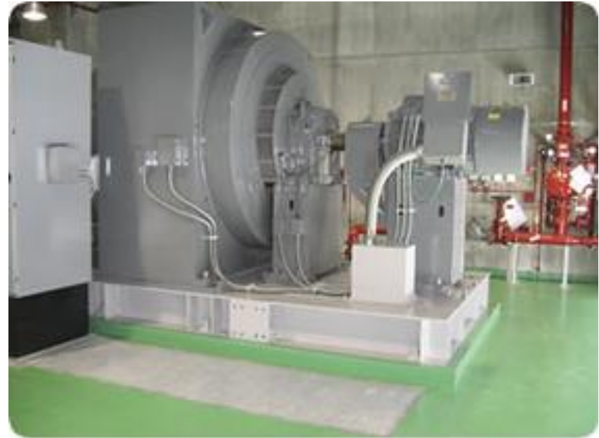
Picture of a synchronous condenser
