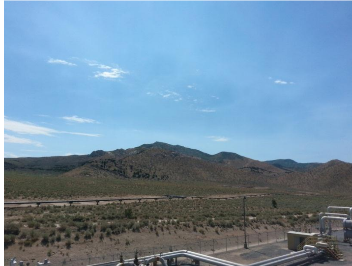
Blundell Geothermal Plant, 33 MW
