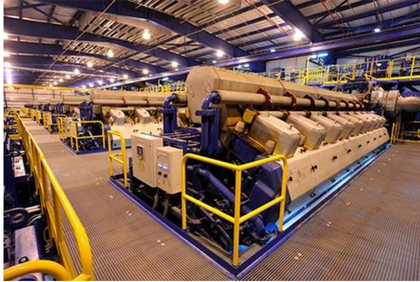
Wartsila 18V50SG engines, 18 MW
