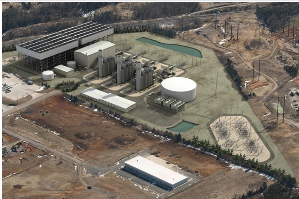
Dominion's Warren County, 3x1 MHI GAC, 1329 MW
