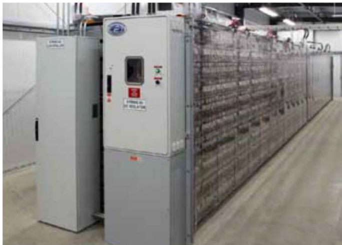
Figure 18 - UberBattery Energy Block
