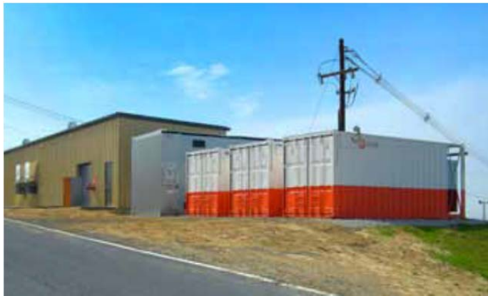
Figure 17 - 3 MW of frequency regulation at the PJM Interconnection
