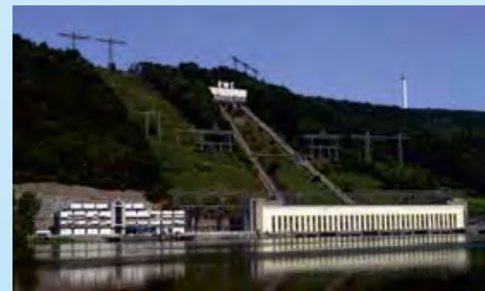
Herdecke pumped-storage power plant
