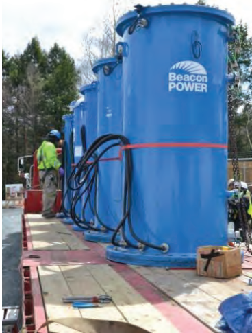
Flywheel assemblies arriving at a plant site
