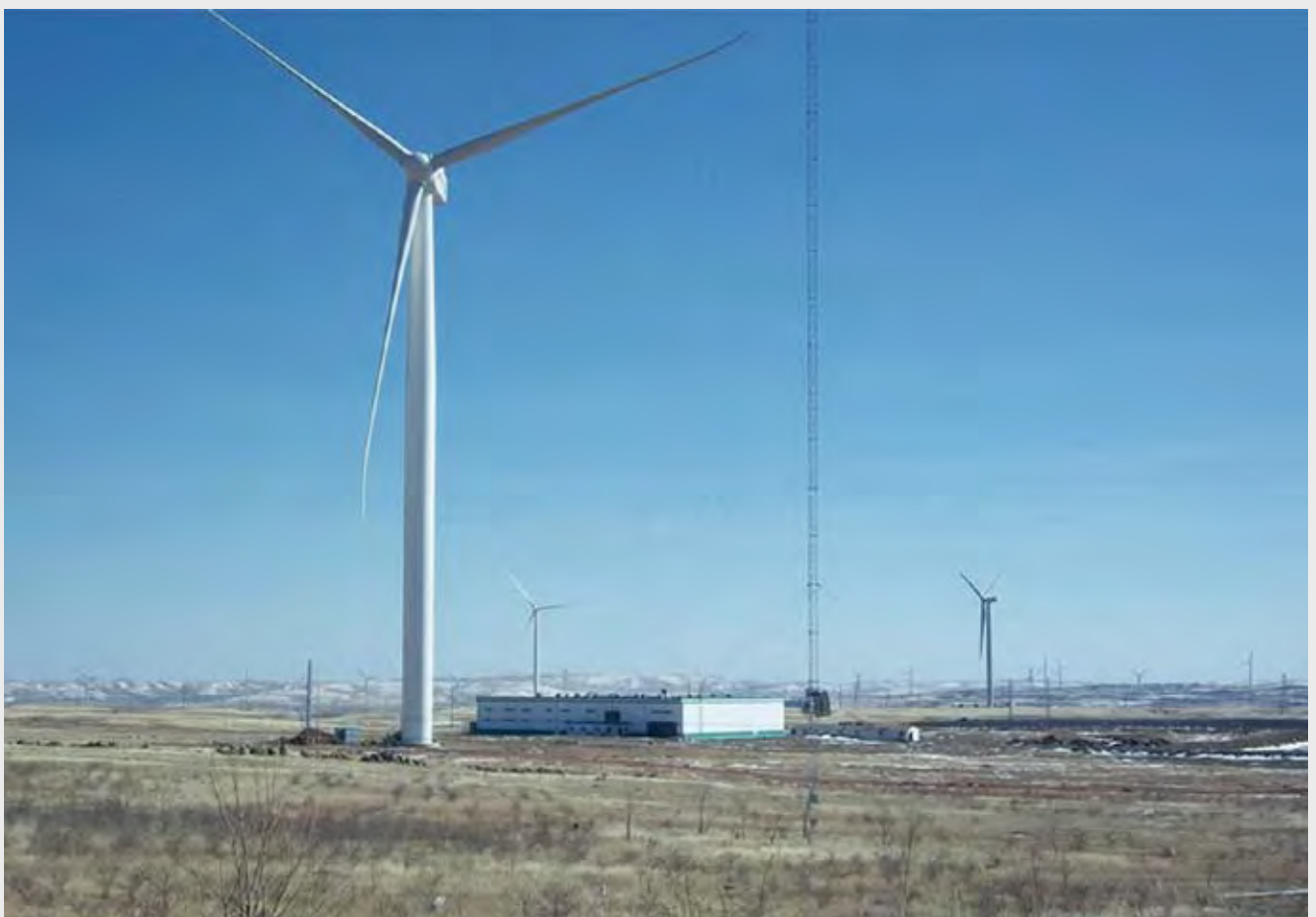
State Grid Project, China
