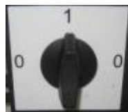
CURRENT TESTING POSITION
