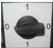
VOLTAGE TESTING POSITION
