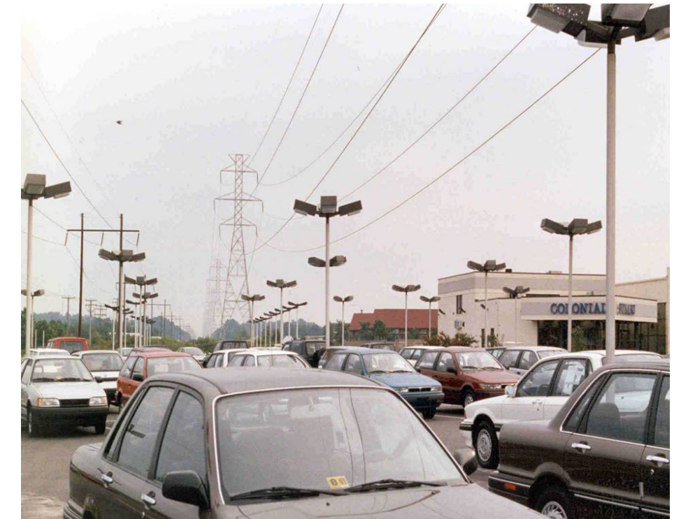
Transmission line running through a large car dealership parking lot
