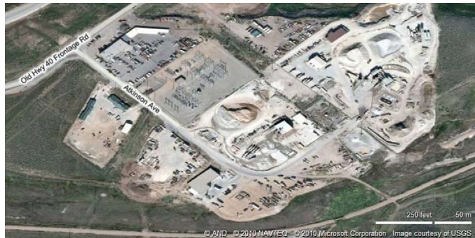
Silver Creek Substation, adjacent to other infrastructure
