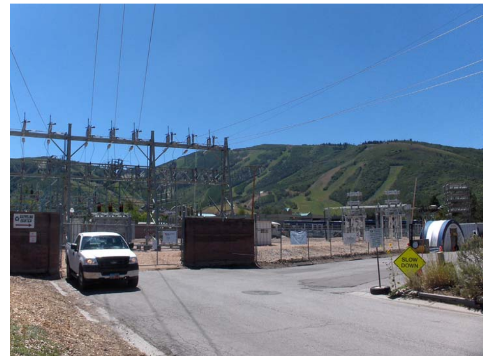
Above: Rose Park Substation 46 kV to 12.5 kV. Below: Park City Substation. 46 kV to 12.5 kV.
