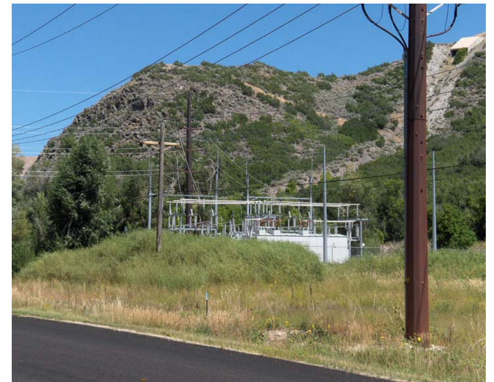
Above: Hammer Substation. 138 kV to 12.5 kV Below: Jordanelle Substation. 138 kV to 12.5 kV.
