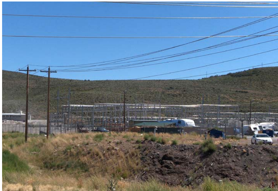
Above: Southeast Substation Regional with Distribution. 138 kV to 12.5 kV Below: Silver Creek Substation 138 kV to 46 kV, 138 kV to 12.5 kV.
