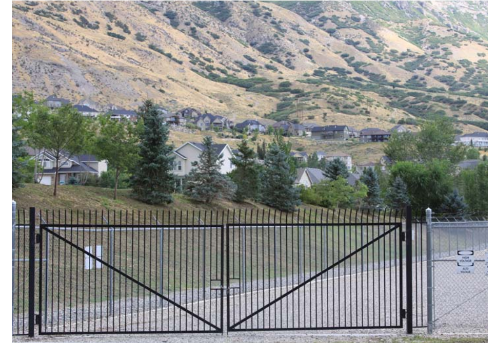
Berms and slopes are used to integrate a substation into the surrounding neighborhood
