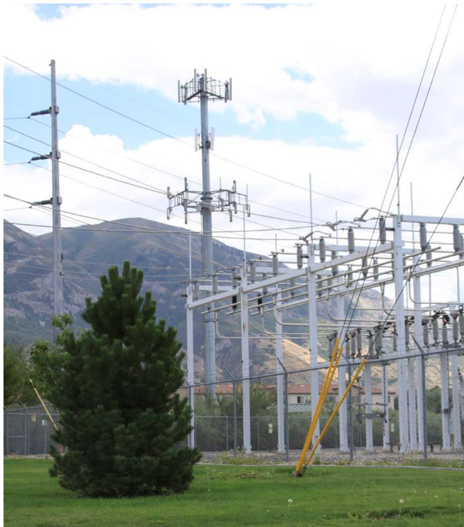
Co-location of telecommunication towers with substations
