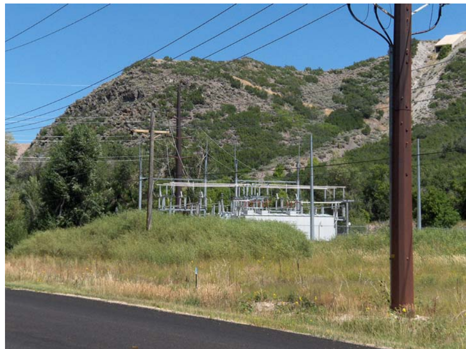
Jordanelle Substation, with a simple fence and landscaping ties into surrounding area
