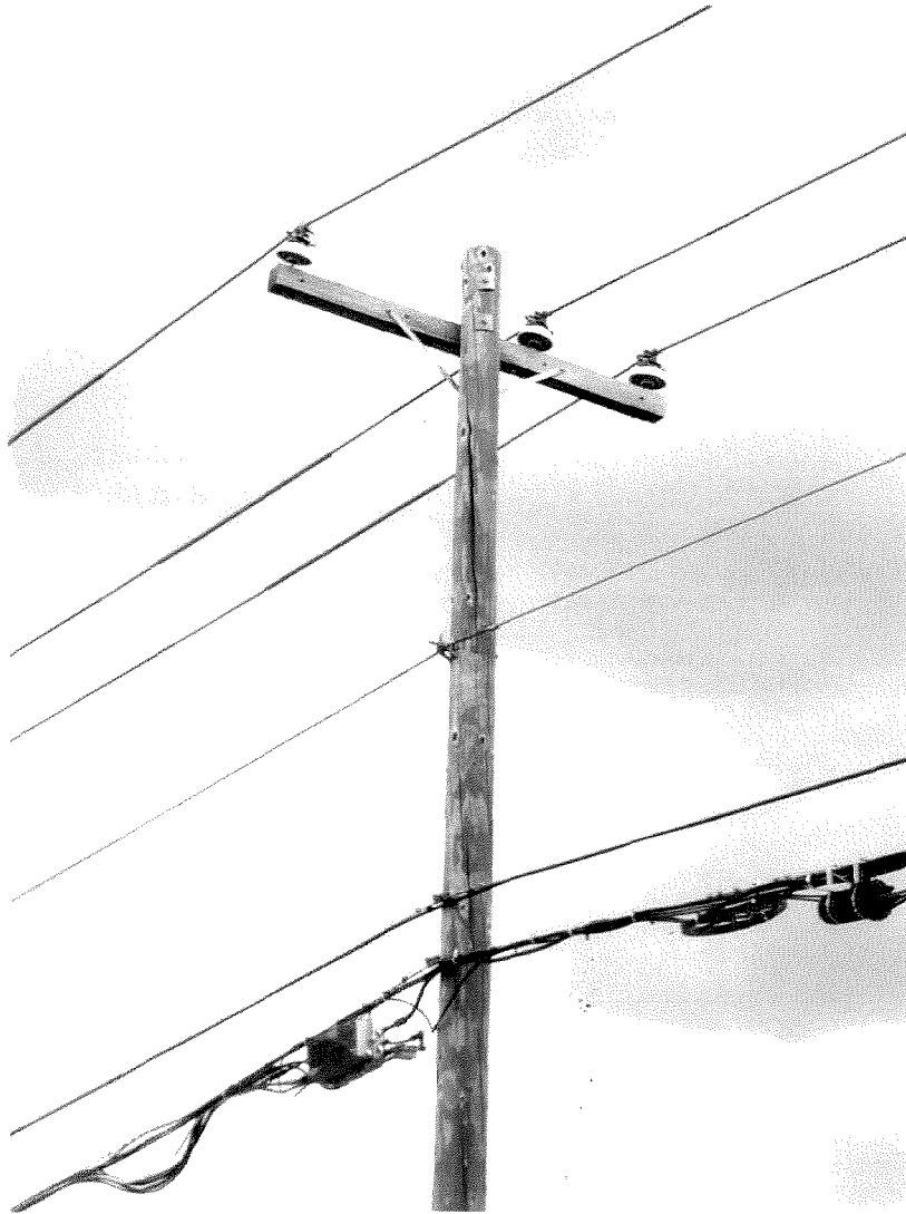
Figure 4—Three-Phase Primary Pole Without Pole-Top Pin Conductor Example
