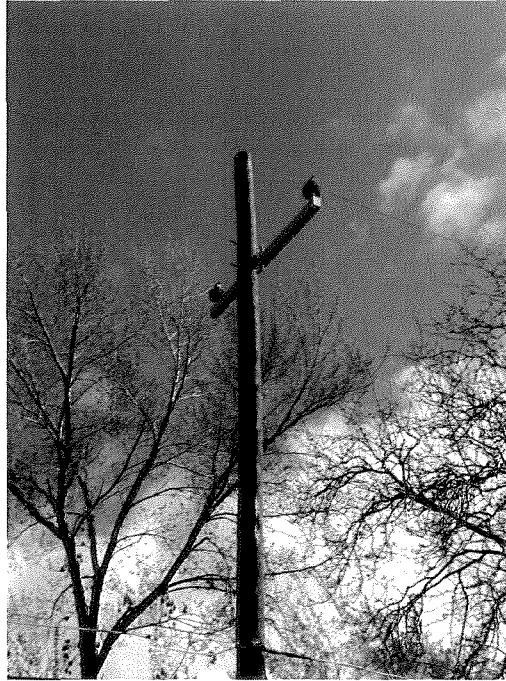
Figure 3—Two-Phase Primary Pole, Example
