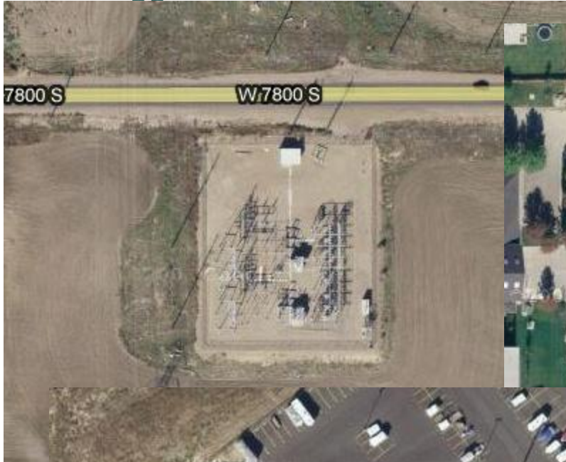
Hoggard substation 138-12.5 kV
