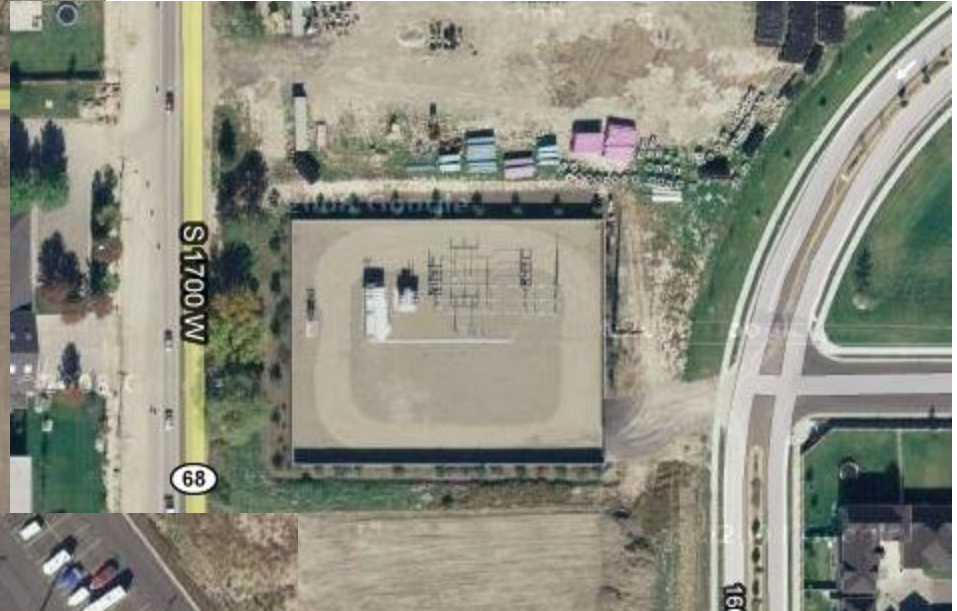
South Jordan substation 138-12.5 kV
