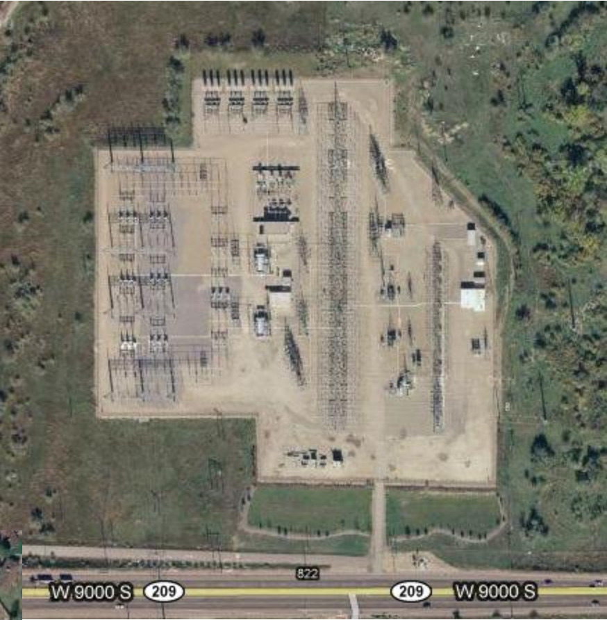
90 th South substation 345-138 kV, 138-46 kV, & 138-12.5 kV
