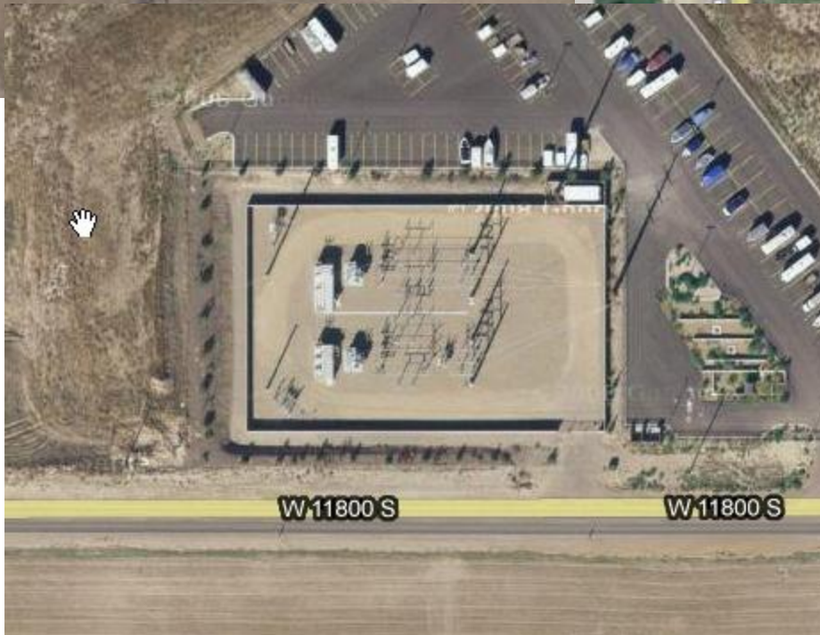
Sunrise substation 138-12.5 kV
