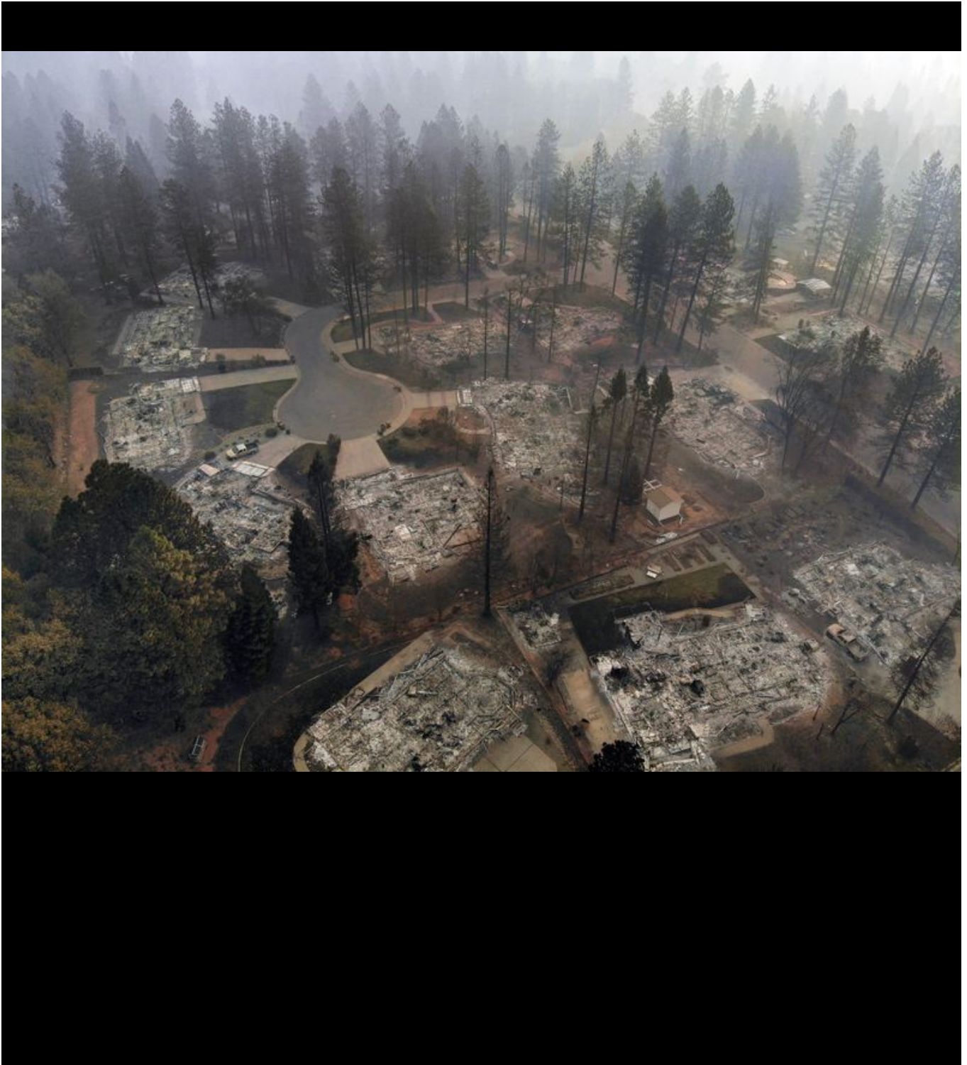
Aerial view of destruction from the Camp fire in Paradise off of Clark Road. The Camp Fire has burned more than 7,000 structures in Paradise. (Carolyn Cole / Los Angeles Times)
