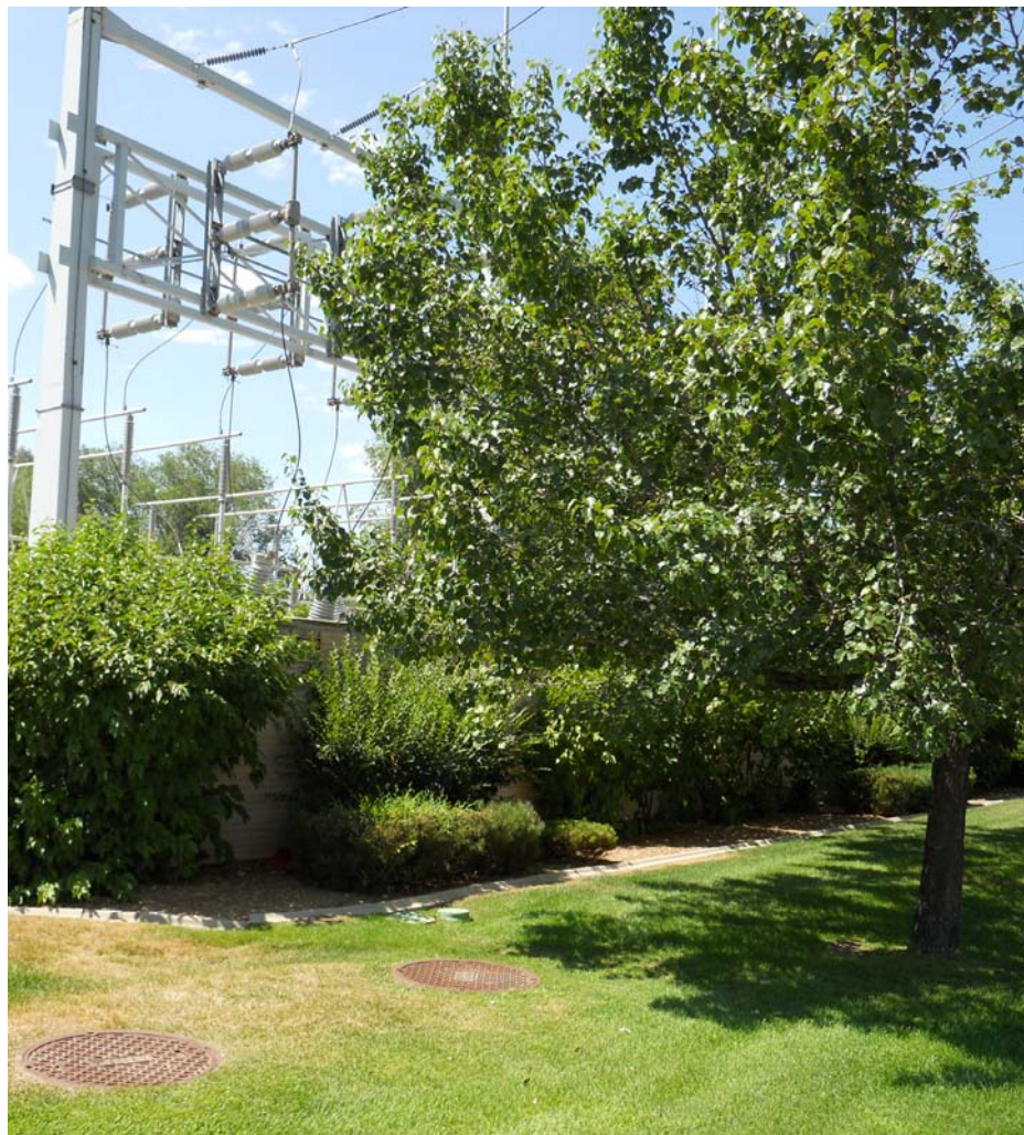
Vegetation acts as a buffer between a substation and the surrounding neighborhood
