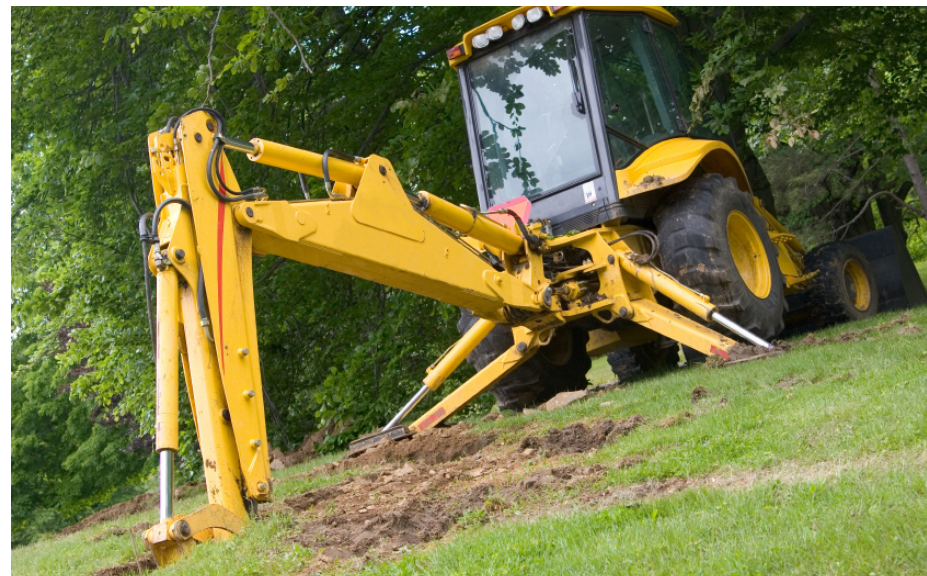
Exercise care during construction to protect vegetation
