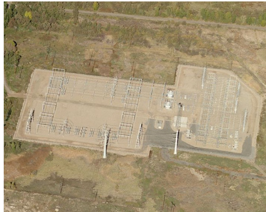
Midvalley Substation. 345 kV to 138 kV
