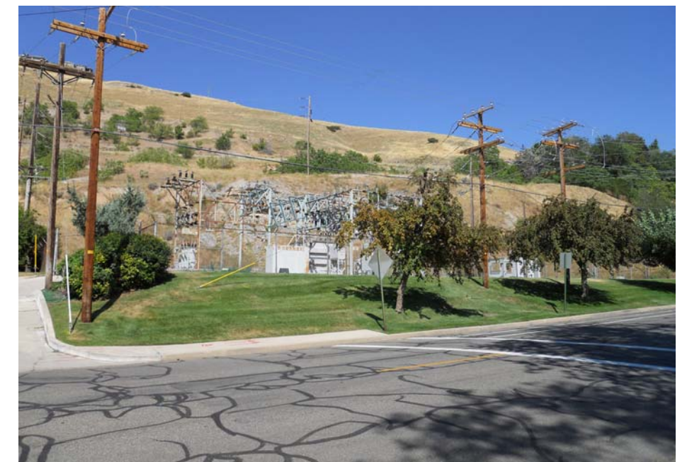
Capitol Substation, 46kV, ties into the quiet neighborhood with a fence and simple landscaping
