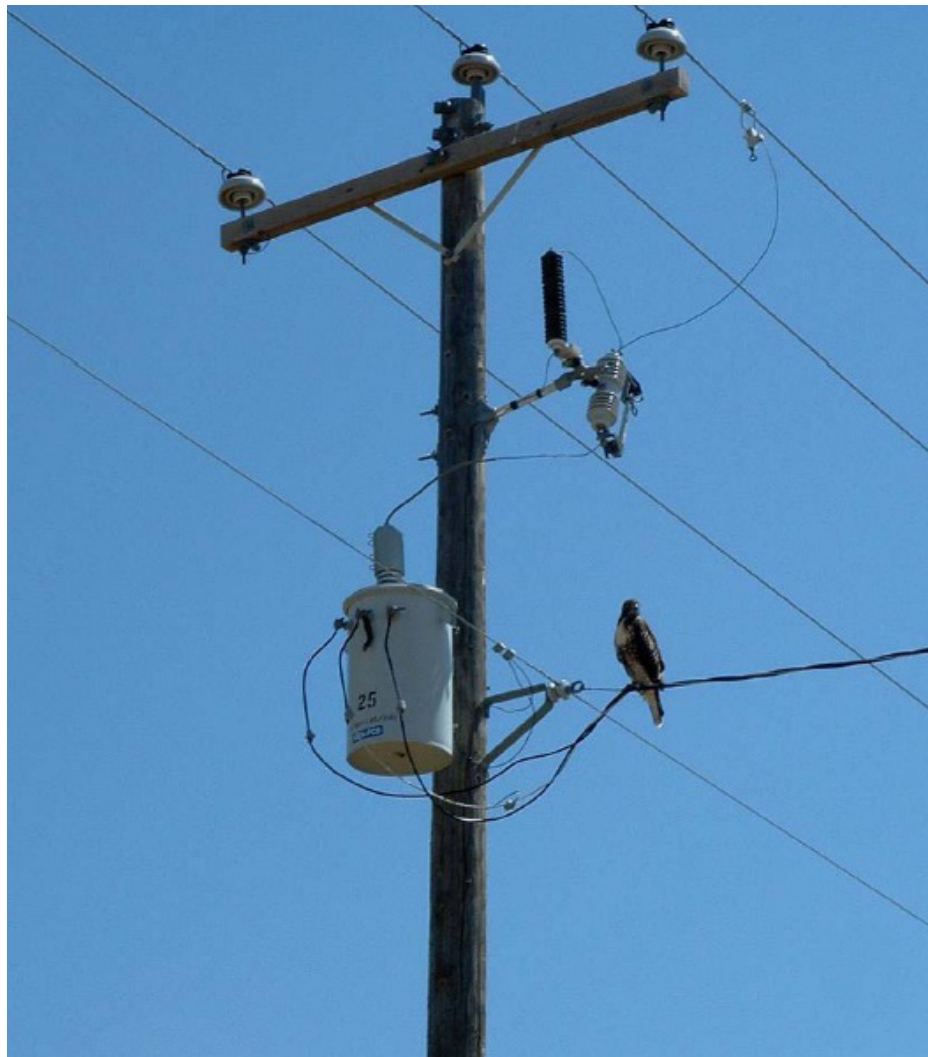
Typical distribution pole
