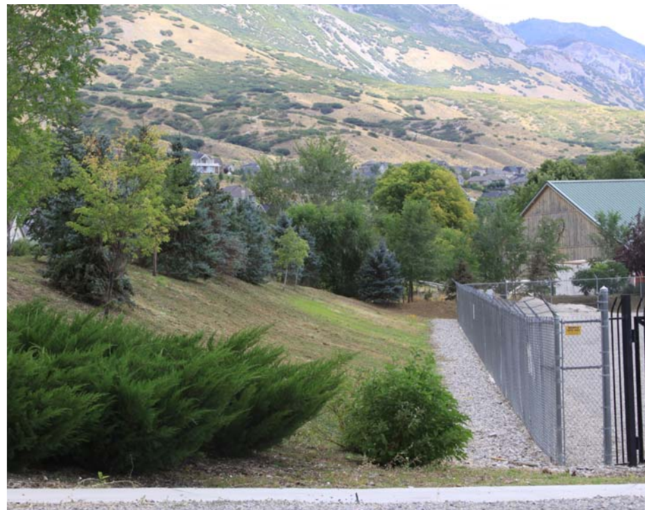
A natural slope obscures the view of a substation to the surrounding neighborhood
