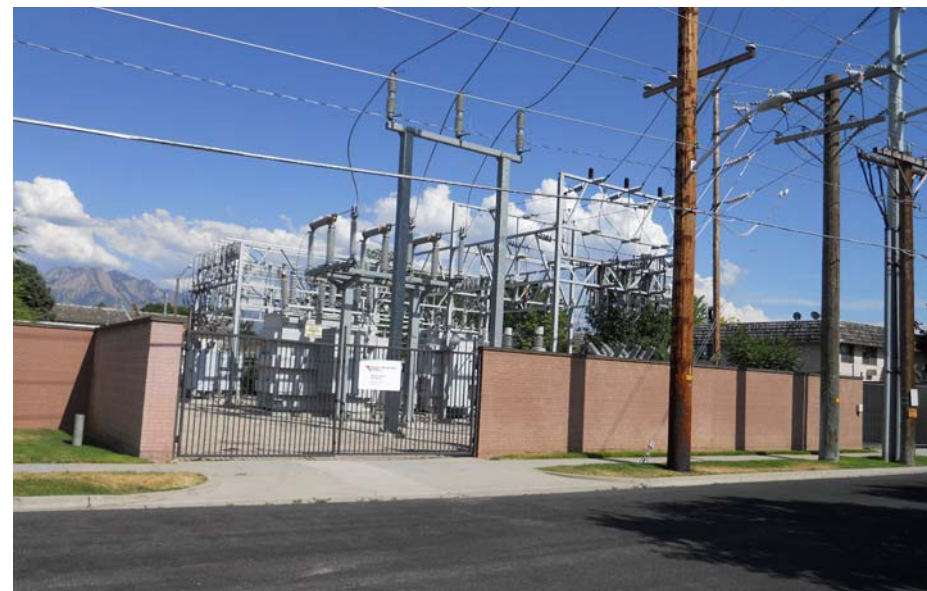
Above: Meadowbrook Substation aerial view. Below: Meadowbrook Substation street view. 138 kV to 12.5 kV.
