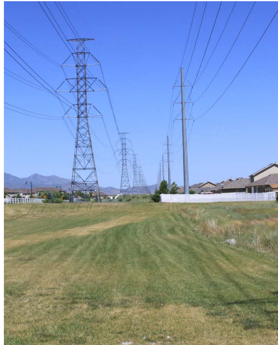
A transmission line utilizes natural green space in order to avoid areas with greater impact
