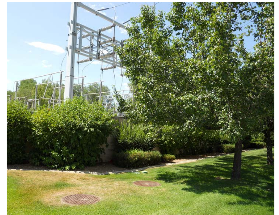
Above: Hammer Substation aerial view. Below: Hammer Substation street view. 138 kV to 12.5 kV.
