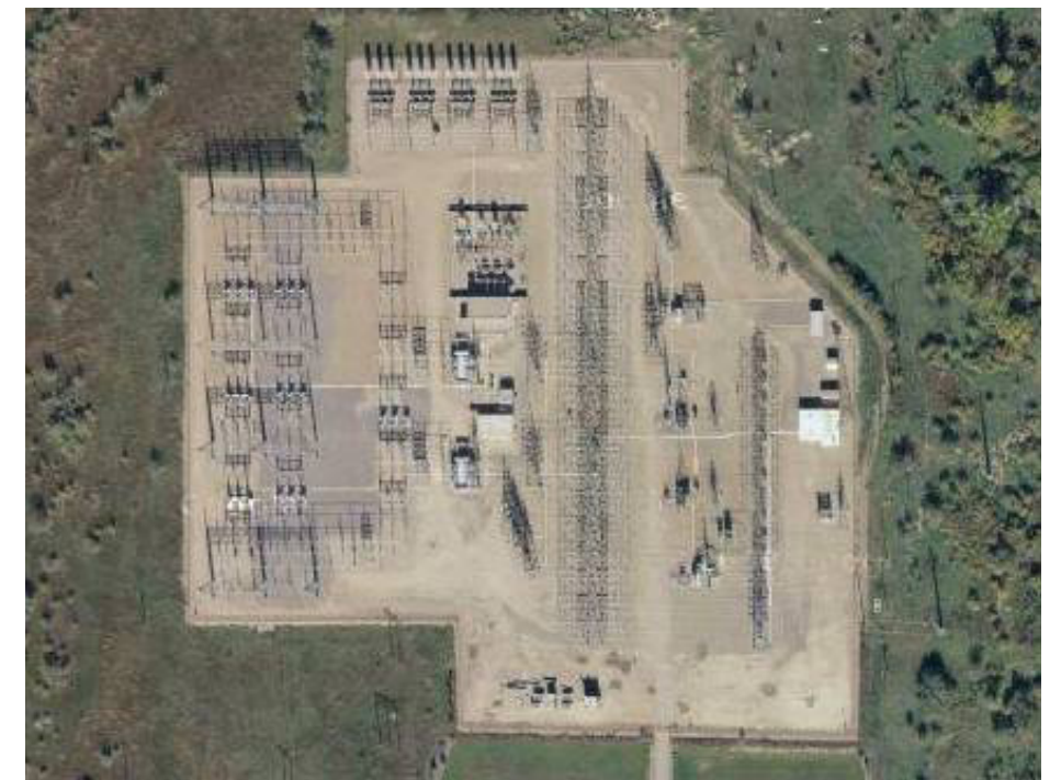
Above: Camp Williams Substation. 345 kV to 138 kV, 138 kV to 46 kV, 138 kV to 12.5 kV. Below: 90th South Substation 345 kV to 138 kV, 138 kV to 46 kV, 138 kV to 12.5 kV.
