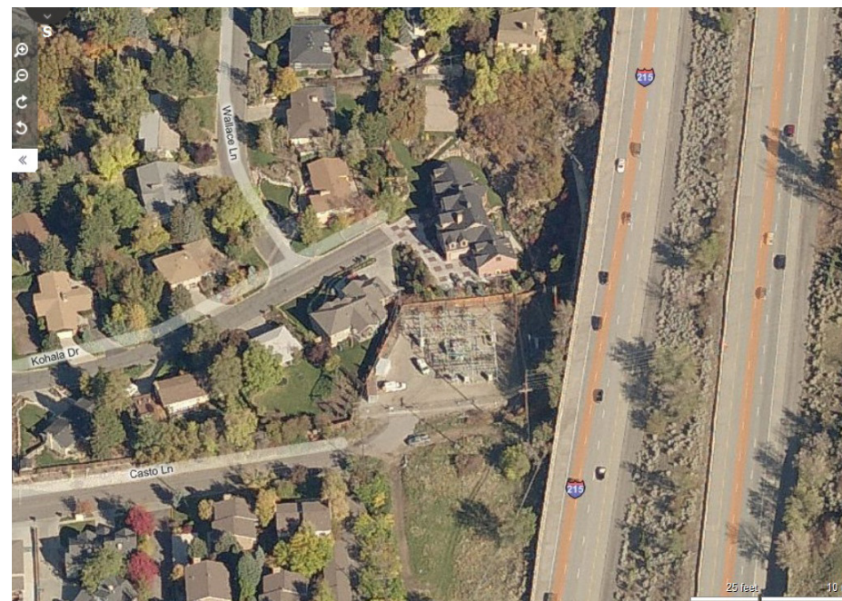
Casto Substation adjacent to Interstate 215
