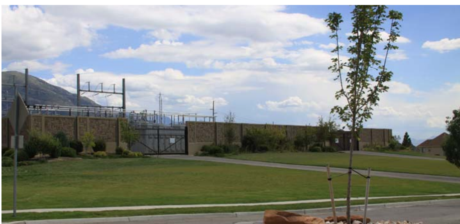
Standard concrete wall with landscaping
