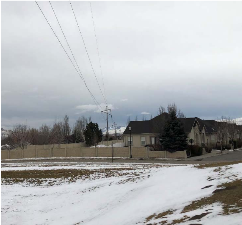
Looking south in South Jordan from 10760 South near 1600 West
