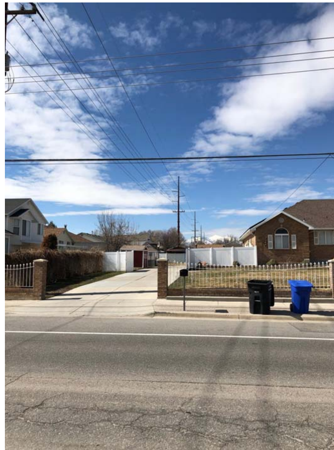
Existing 46 kV single circuit
