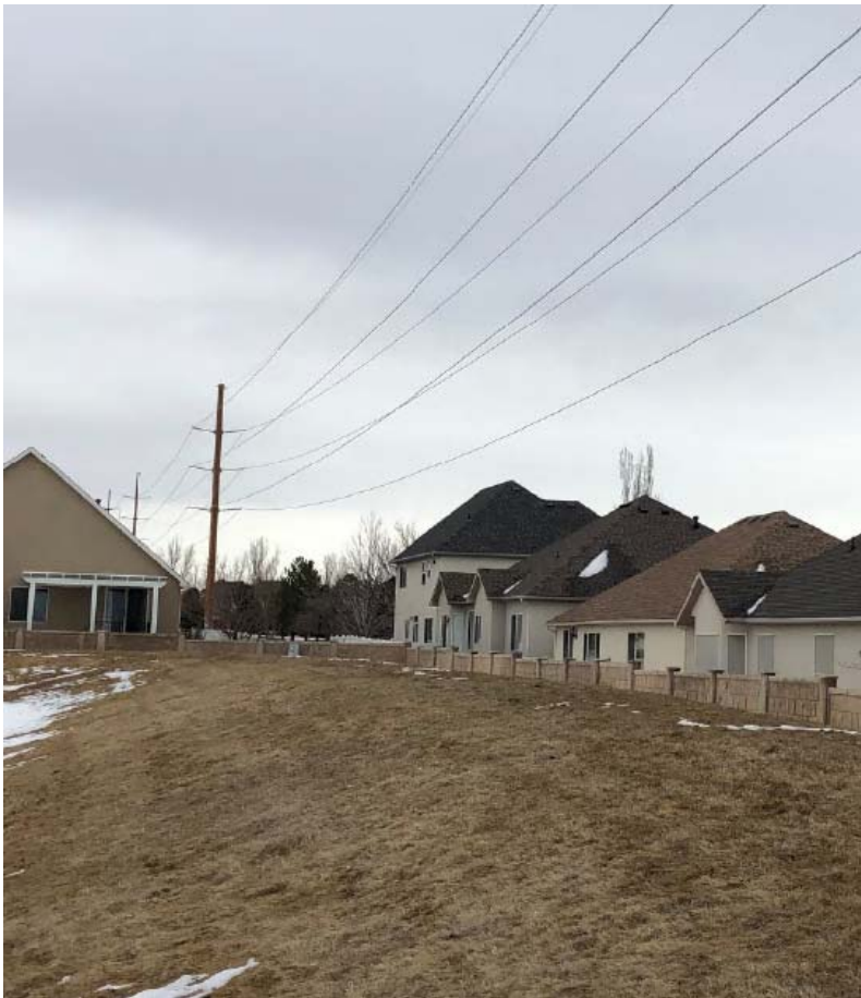
Existing 46 kV and 138 kV double circuit
