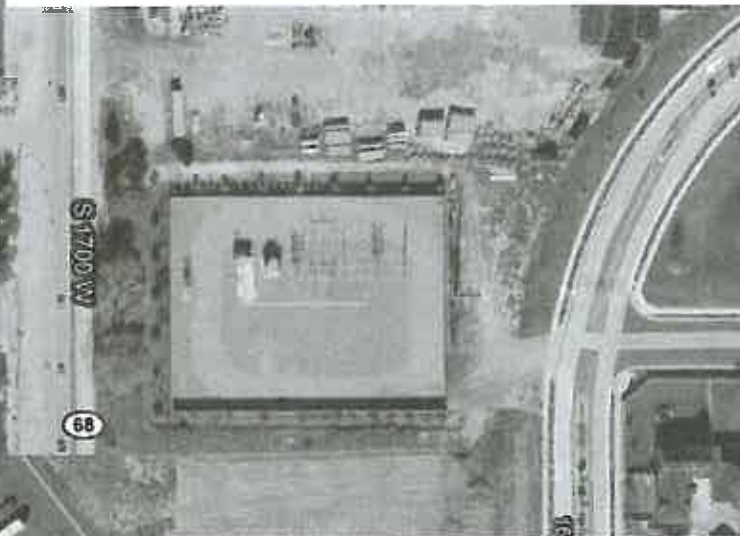
South Jordan substation 138-12.5 kV
