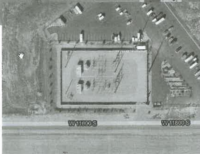
Sunrise substation 138-12.5 kV
