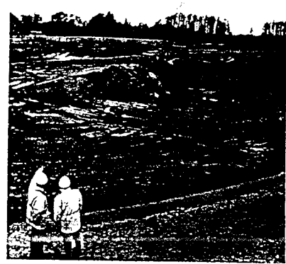
New reservoir under construction at Testwood Lakes.
