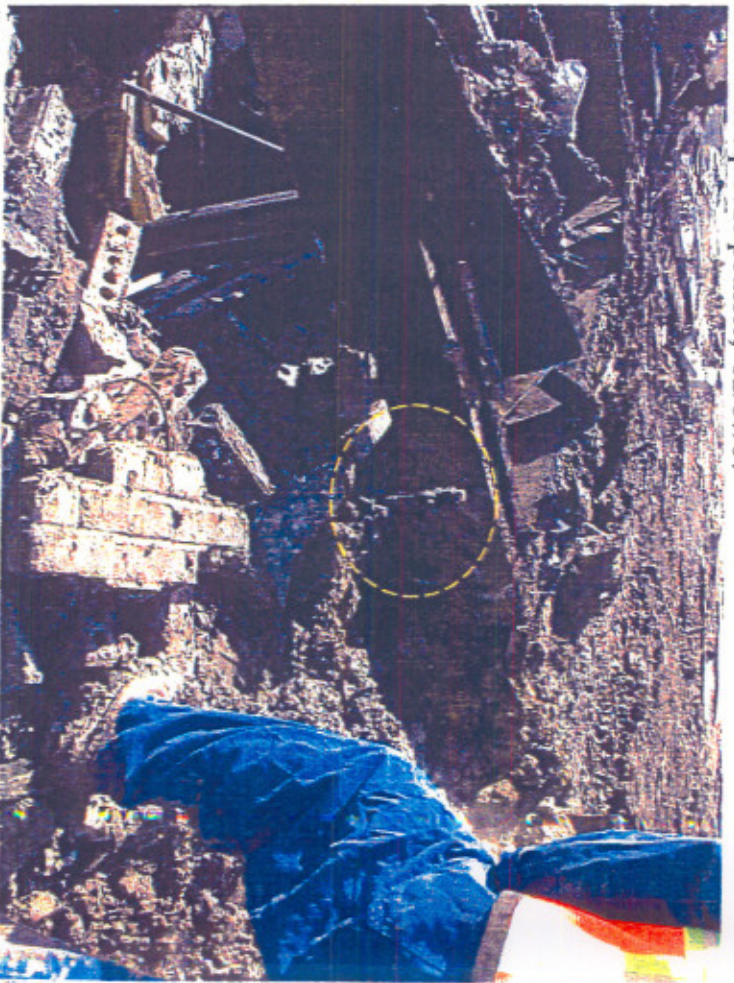
#16 East side of main, N.W. corner, 02/07/07
