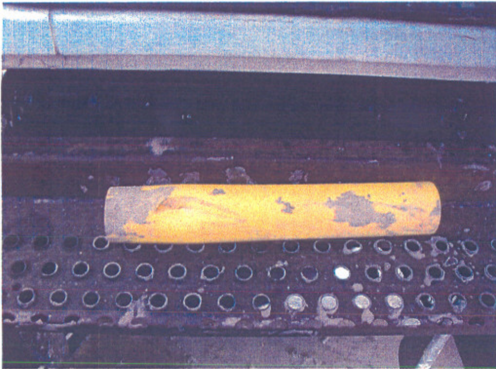
#29 Damaged section of the main, 02/07/07
