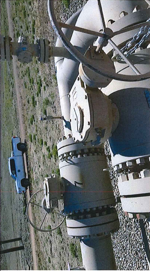
Picture #17: Observed pig launcher with BV-7 and BV-8 in the close position and BV-5 in the open position. All valves chained and locked.
