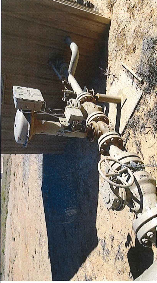
Picture #10: Block Valve BV-10, observed in open position with chain and lock.
