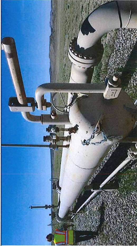
Picture #17: Observed pig launcher with BV-7 and BV-8 in the close position and BV-5 in the open position. All valves chained and locked.
