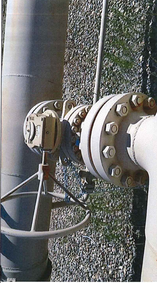
Picture #18: Block Valve BV-6, observed in close position with chain and lock.
