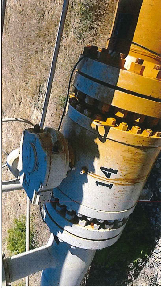
Picture #5: Block Valve BV-14 south side, observed in open position with chain and lock.
