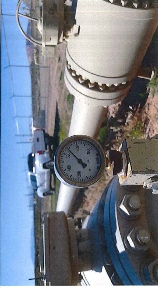
Picture #2: Pressure gauge near BV-18, observed pressure in pipeline, approximately 680 psig.
