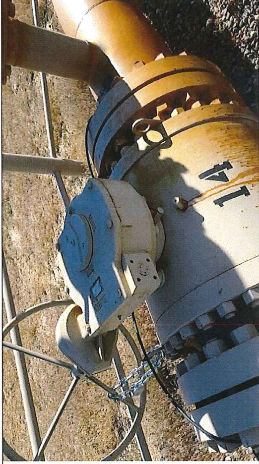
Picture #5: Block Valve BV-14 south side, observed in open position with chain and lock.
