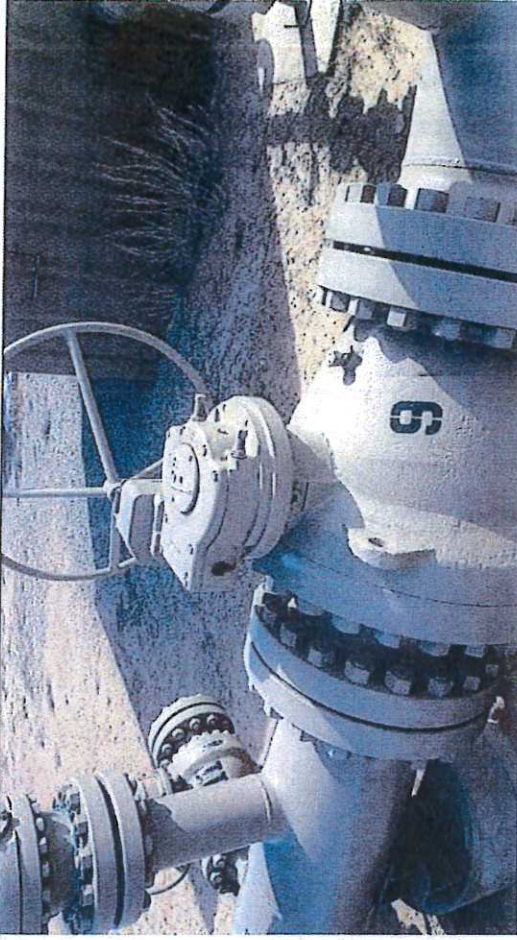
Picture #11: Block Valve BV-9, observed in close position with chain and lock.
