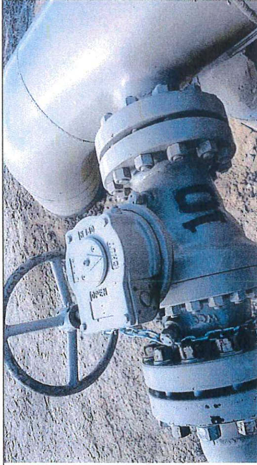
Picture #12: Block Valve BV-10, observed in close position with chain and lock.
