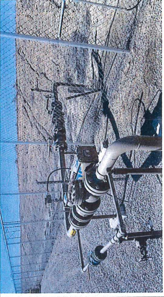
Picture #14: Observed Wesco Compressor Station at Blue Hills pressure gauge approximately 680 psig.
