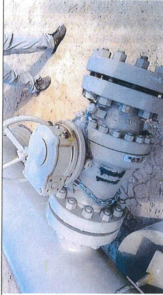
Picture #11: Block Valve BV-9, observed in close position with chain and lock.
