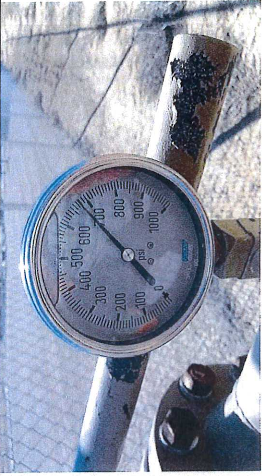
Picture #14: Observed Wesco Compressor Station at Blue Hills pressure gauge approximately 680 psig.
