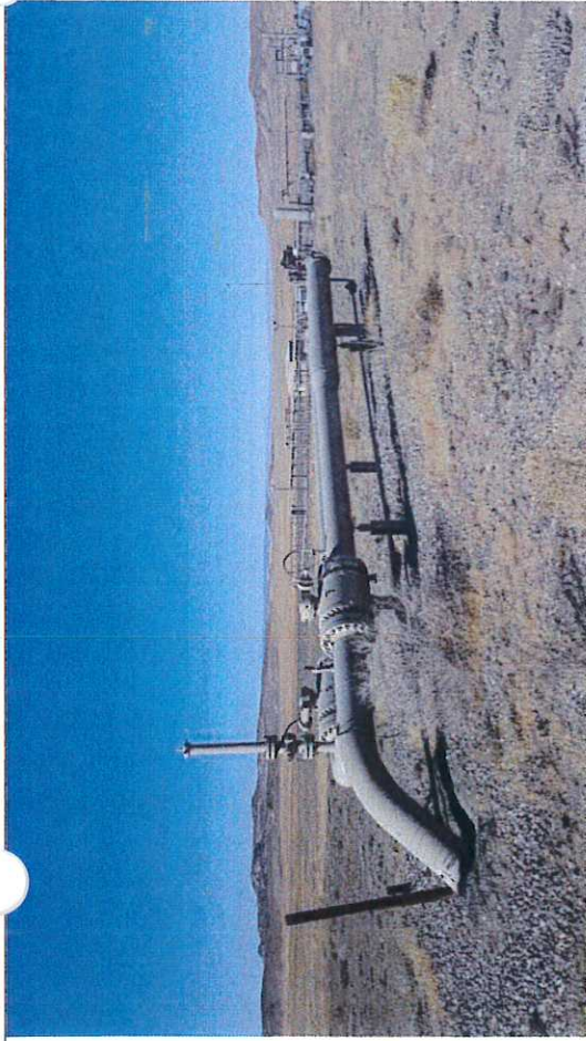
Picture #28: Observed PEMC pig launcher.
