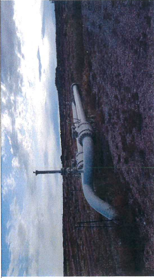
Picture #1: PEMC Pig Receiver near Williams Tap.
