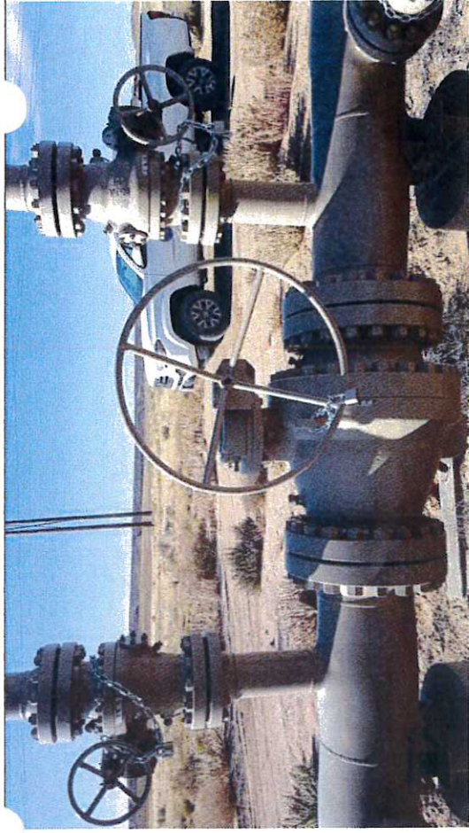
Picture #19: Behind Block Valve BV-9, BV-12 and BV-13, observed in close position with chain and lock.
