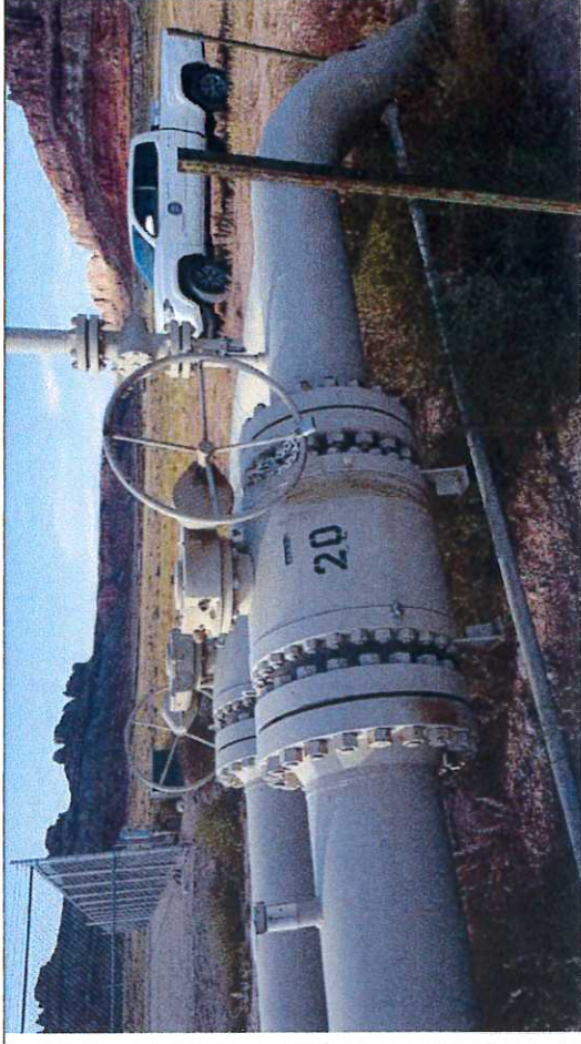
Picture #2: Block Valve BV-21, observed in close position with chain and lock.
