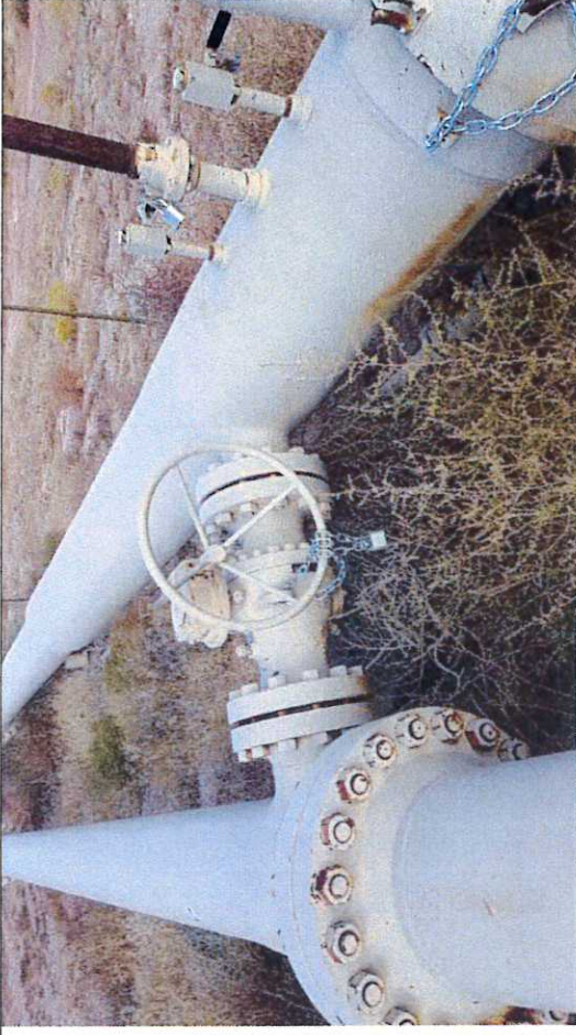
Picture #2: Block Valve BV-21, observed in close position with chain and lock.
