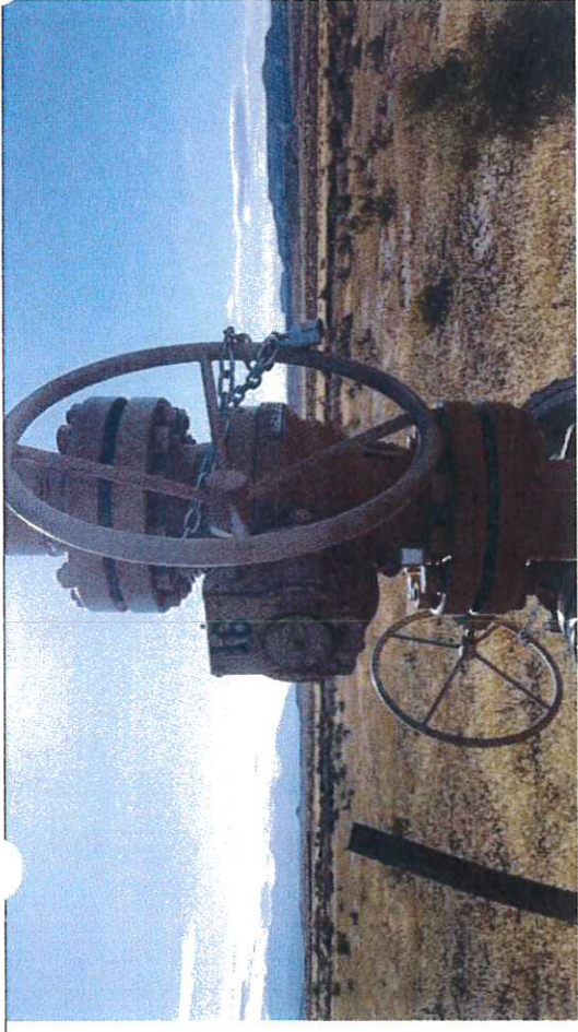
Picture #13 Block Valve BV-16, observed in close position with chain and lock.
