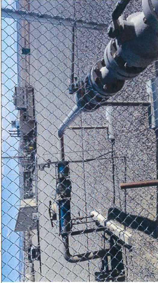
Picture #24: Observe Wesco Compressor Station at Blue Hills, PEMC Valve open position.
