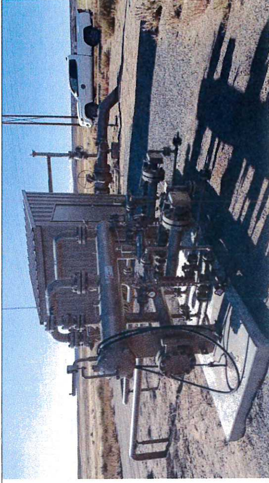
Picture #19: Behind Block Valve BV-9, BV-12 and BV-13, observed in close position with chain and lock.
