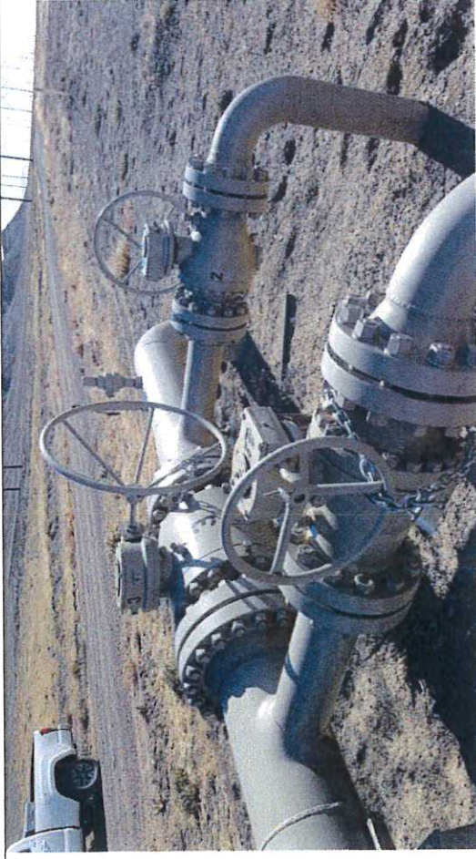
Picture #38: Block Valve BV-3, observed in close position with chain and lock.
