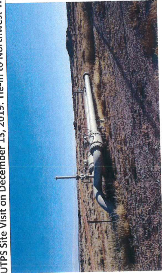
Picture #1: PEMC Pig Receiver near Williams Tap.
