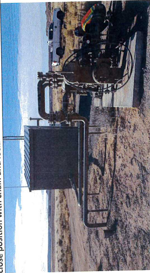
Picture #18: Block Valve BV-10, observed in close position with chain and lock.
