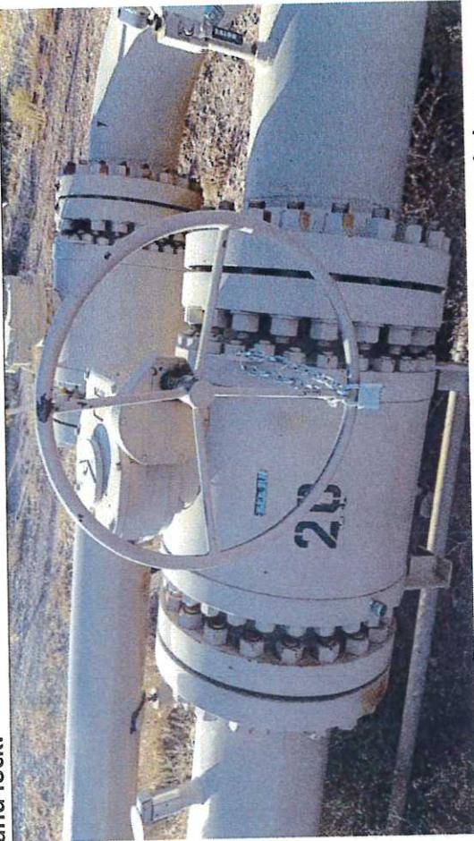
Picture #2: Block Valve BV-21, observed in close position with chain and lock.
