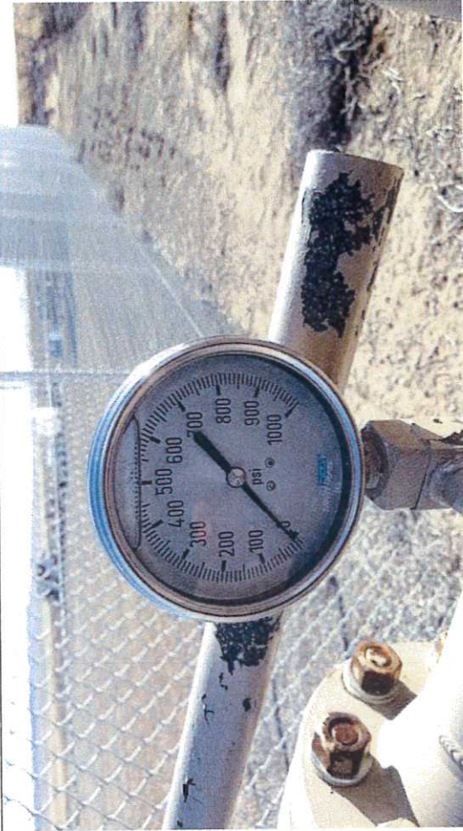
Picture #25: Observed Wesco Compressor Station at Blue Hills pressure gauge approximately 0 psig.
