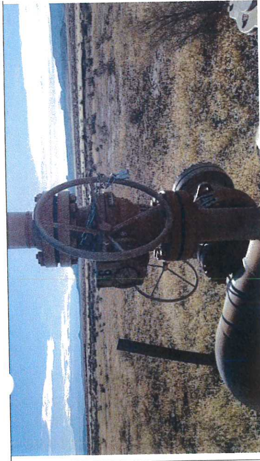
Picture #13 Block Valve BV-16, observed in close position with chain and lock.
