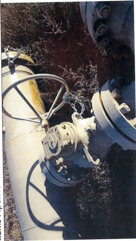
Picture #2: Block Valve BV-21, observed in close position with chain and lock.
