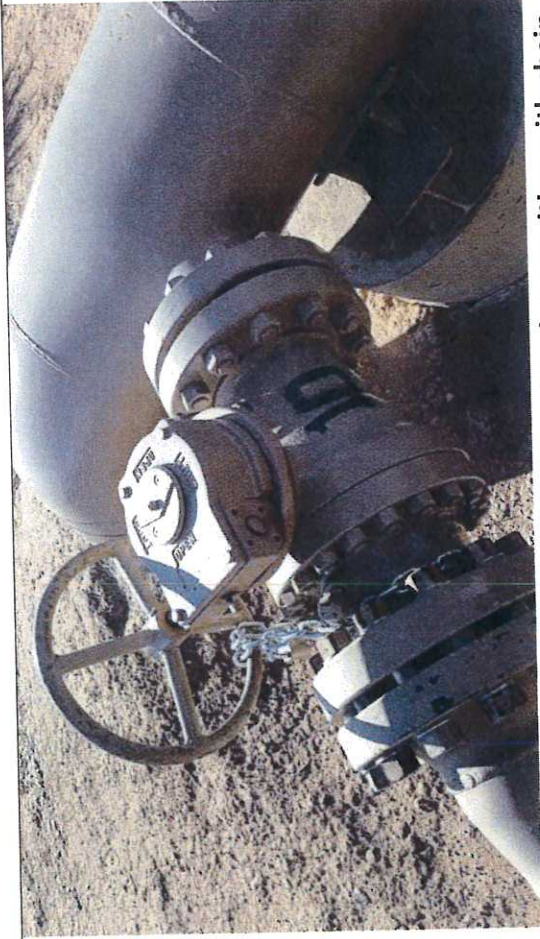
Picture #17: Block Valve BV-11, observed in close position with chain and lock.
