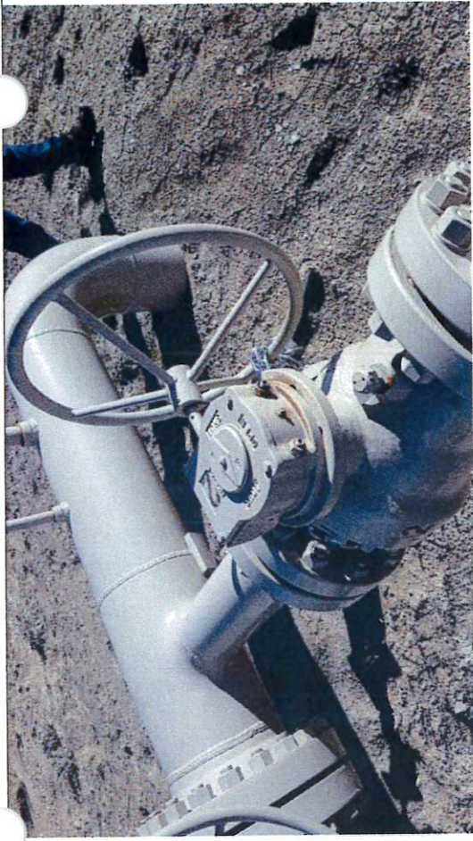
Picture #39: Block Valve BV-2, observed in close position with chain and lock.
