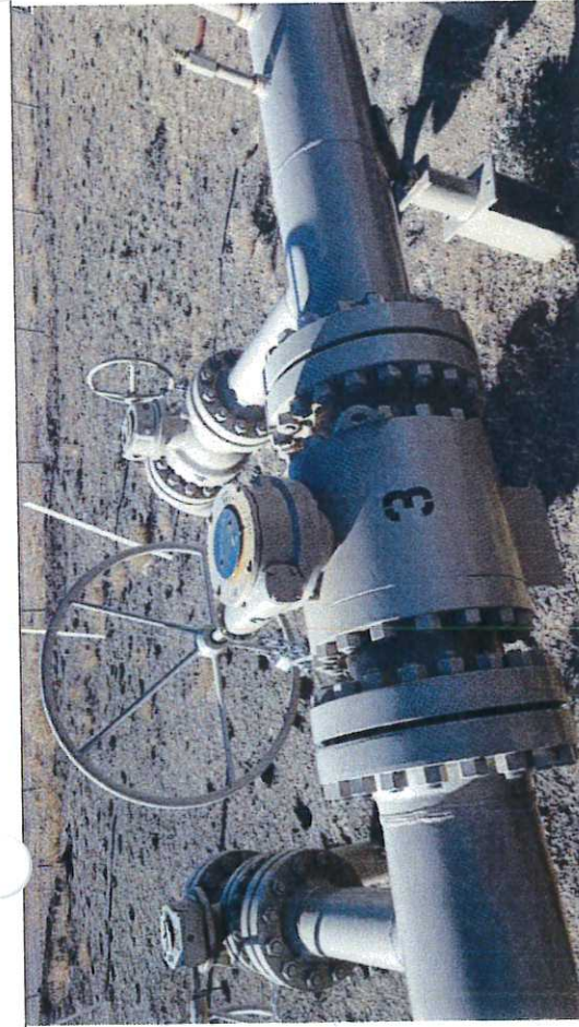
Picture #38: Block Valve BV-3, observed in close position with chain and lock.
