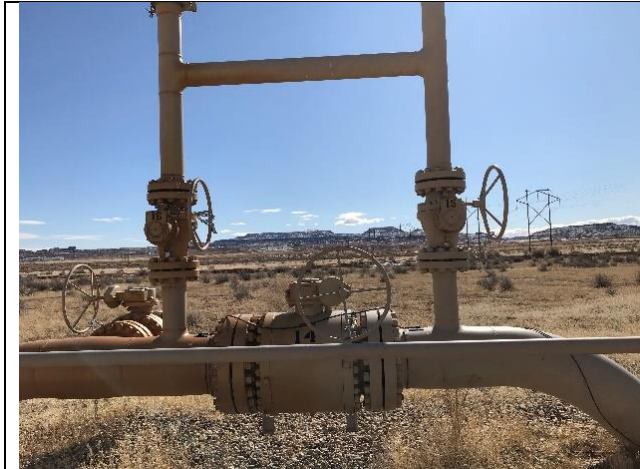
P19. Block valve assembly southwest of the Moab airport.
