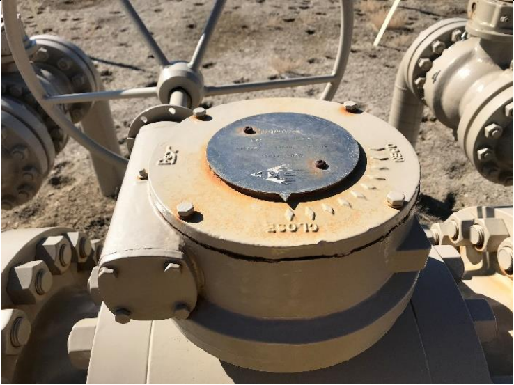
P4. Top of BV#3 indicated closed position.
