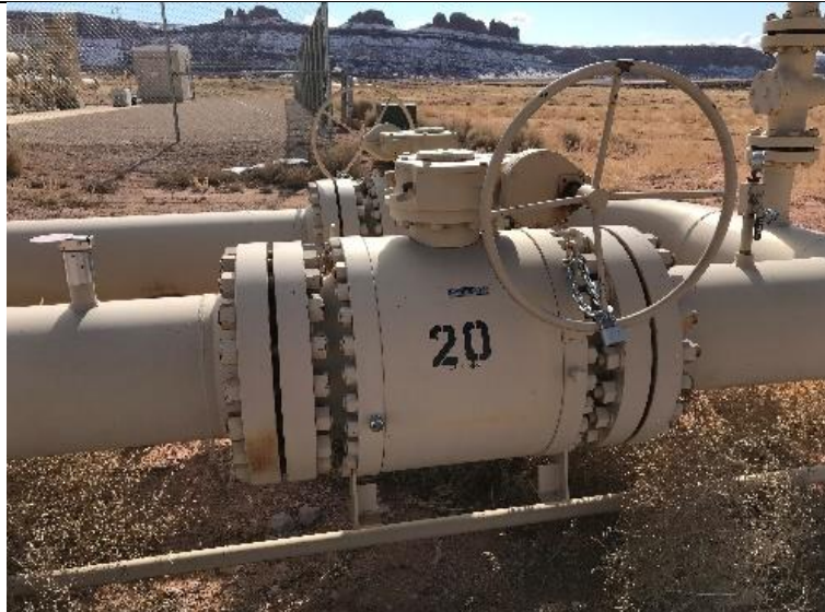
P28. V#20 – Chained and locked in closed position.
