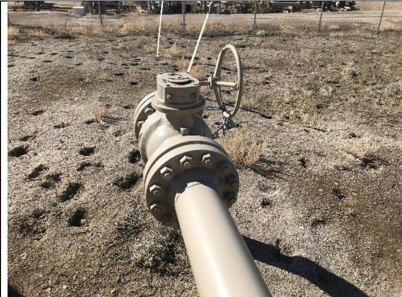
P5. V#2 - Chained and locked in closed position.
