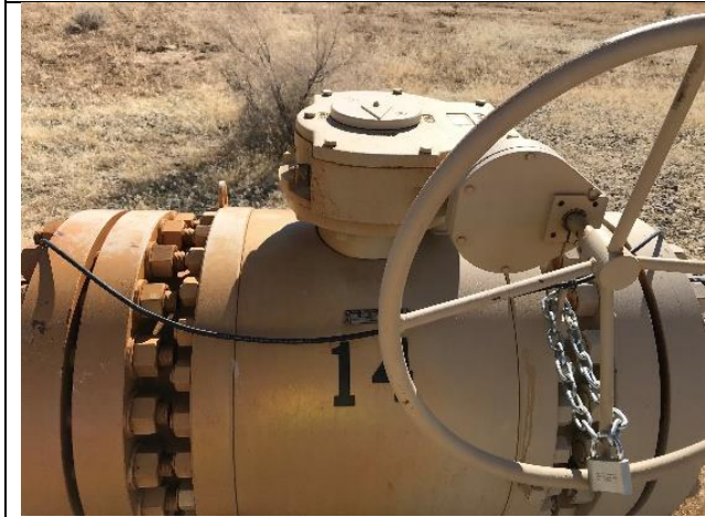
P21. Valve position indicator on BV#14 shows closed position.
