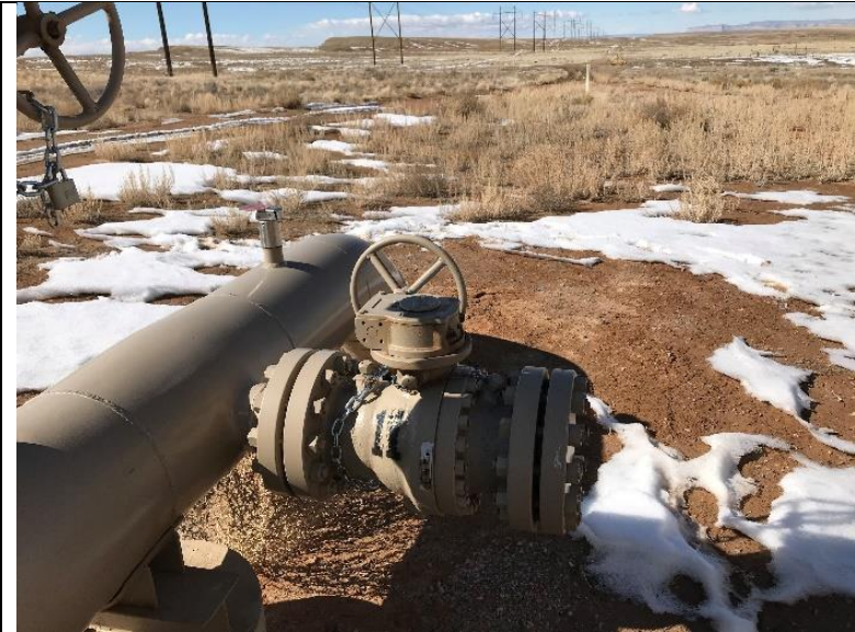
P17. V#11 – Chained and locked in closed position.
