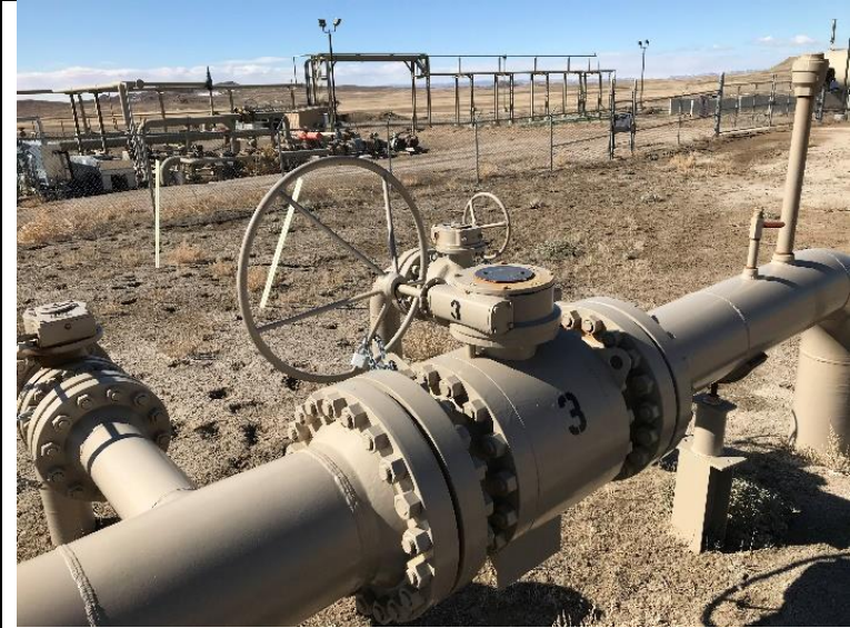
P3. BV#3 - Chained and locked in closed position.
