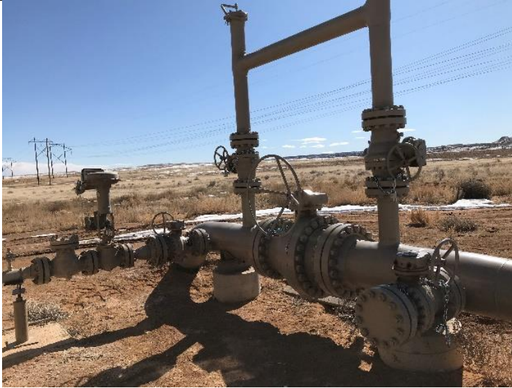
P16. BVs #9, and V#s 10, 11, 12, & 13 – Chained and locked in closed position.
