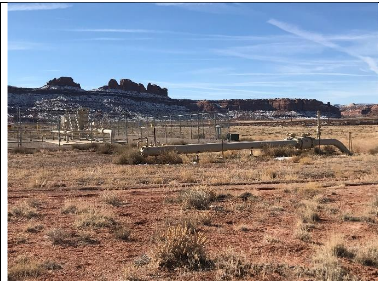
P25. Piping assembly north of NW Williams yard.
