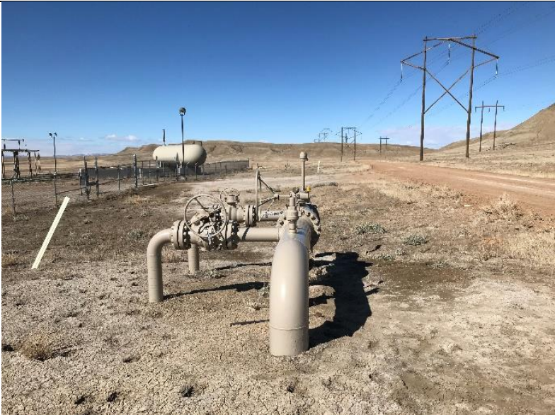
P2. The piping north of PEMC plant: BV#3, and V#s 2 and 4.
