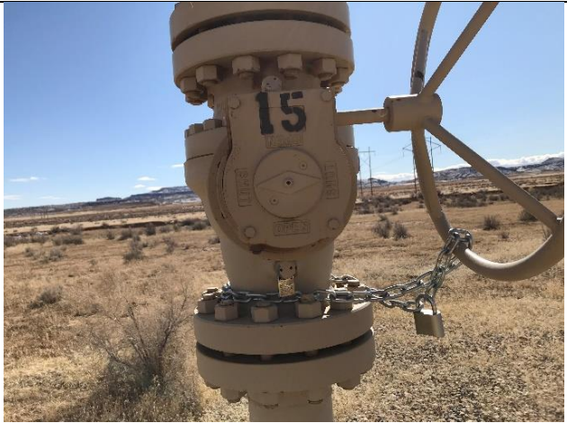
P22. Valve position indicator on V#15 shows closed position.
