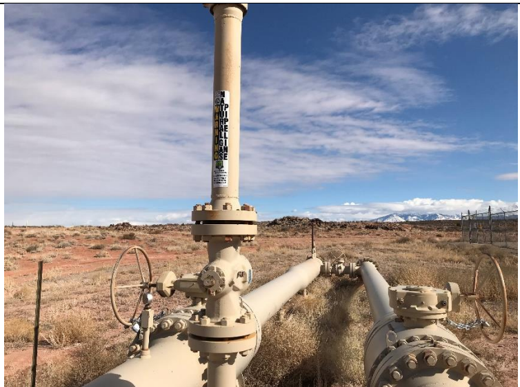
P26. BV# 18 and V#s 19, 20 & 21 – Chained and locked in closed position.
