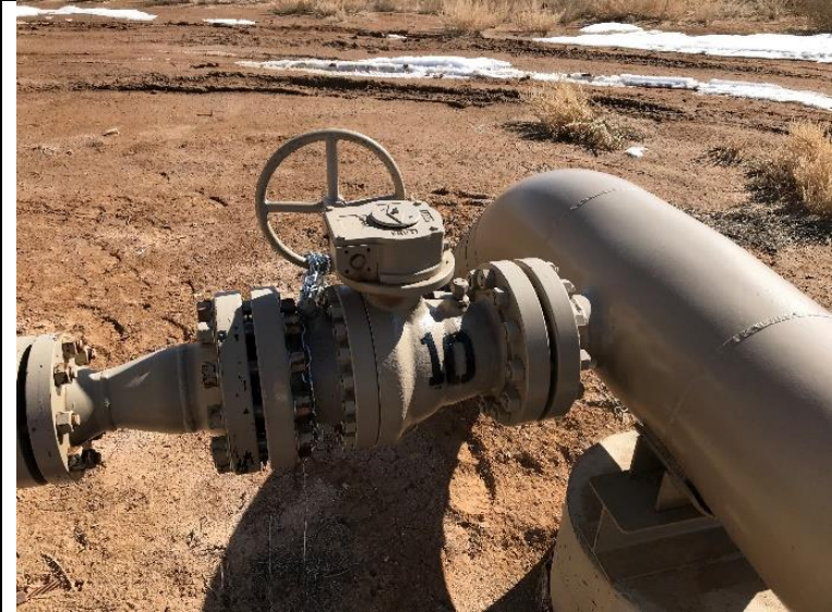
P15. V#10 – Chained and locked in closed position.
