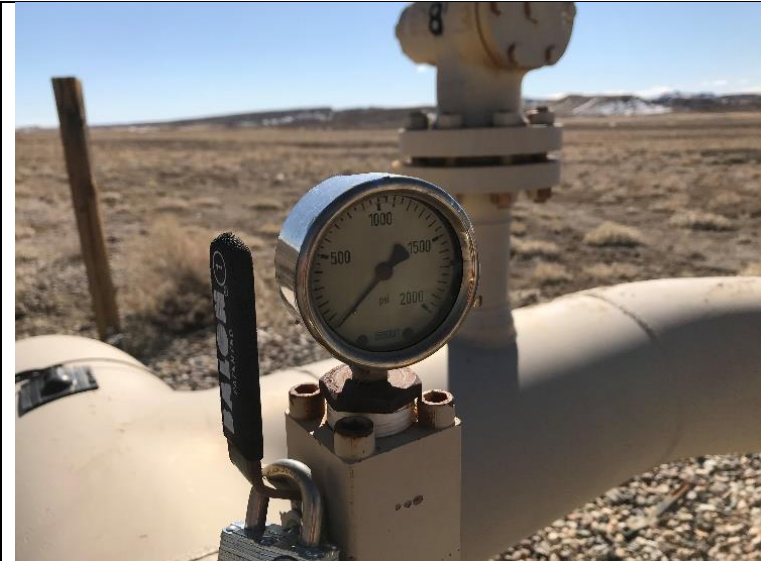
P9. Pressure gauge next to V#7.
