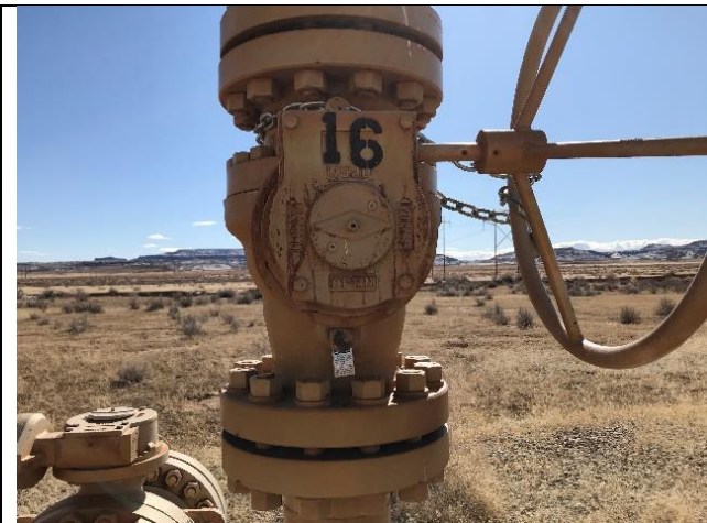
P23. Valve position indicator on BV#16 shows closed position.
