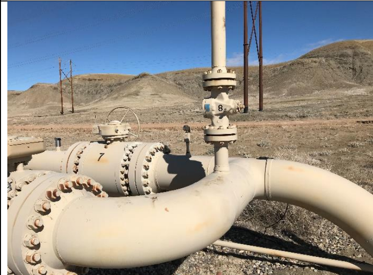
P11. V#7 and vent valve #8 – Chained and locked in closed position.
