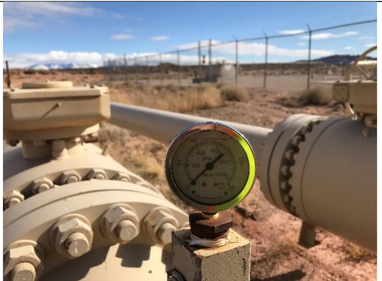
P30. Pressure gauge next to V#20 – indicates zero pressure.
