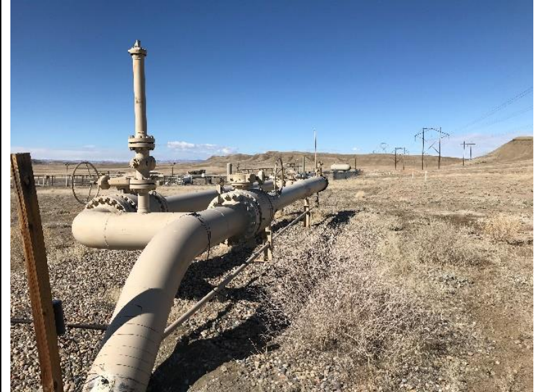
P7. The pig launcher/receiver east of the PEMC plant.
