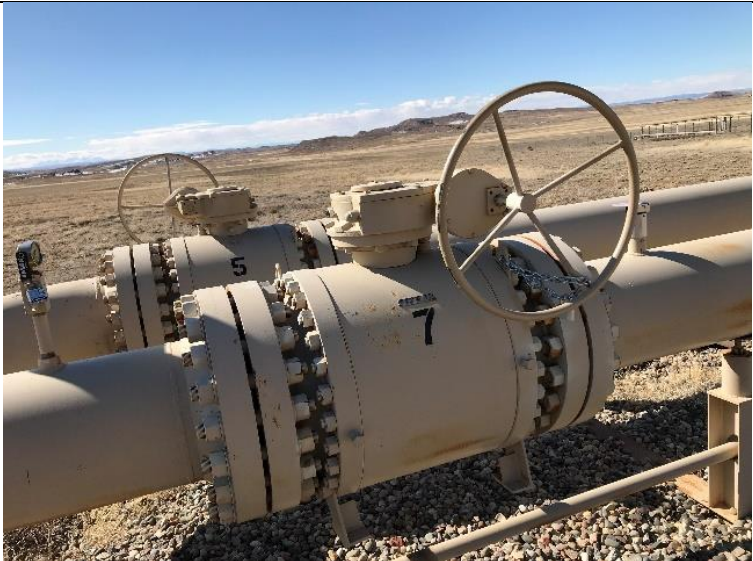
P10. Pressure gauge next to V#7.
