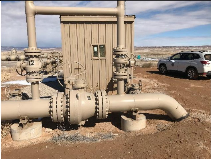
P14. BV#9 and V#s 12 & 13 – Chained and locked in closed position.
