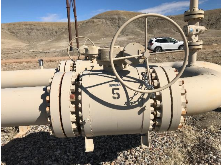
P8. BV#5, and V#s 7 and 8 – Chained and locked in closed position.
