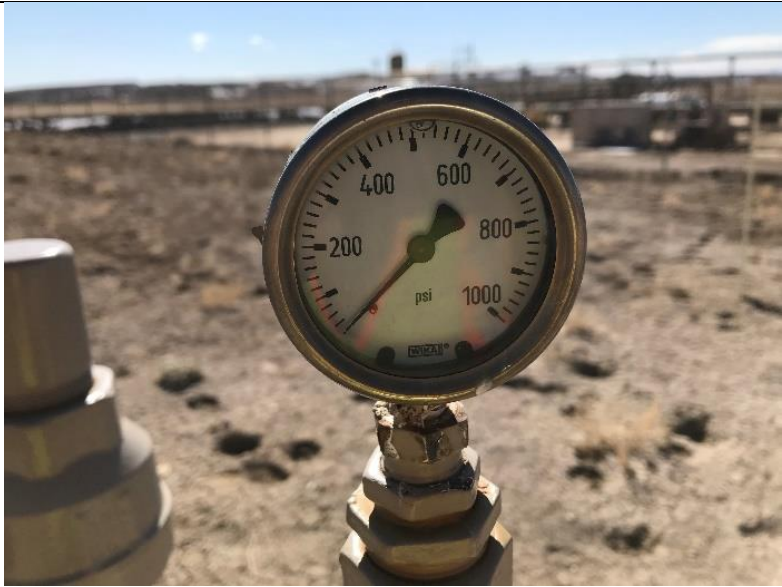
P6. Pressure gauge next to BV#3.
