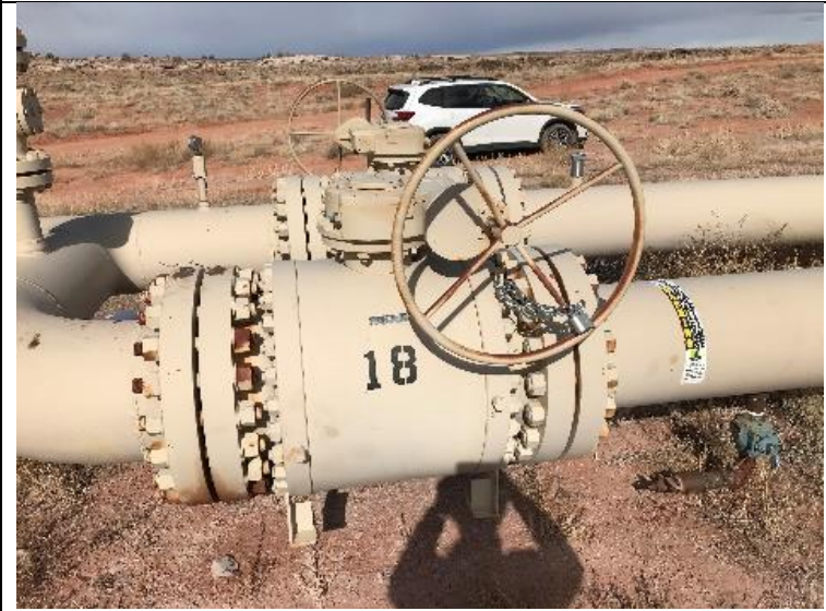
P27. BV#18 – Chained and locked in closed position.
