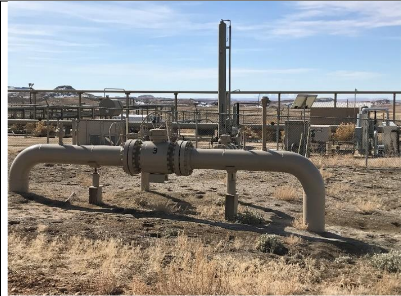
Picture #1. The piping north of PEMC plant: BV#3, and V#s 2 and 4.
