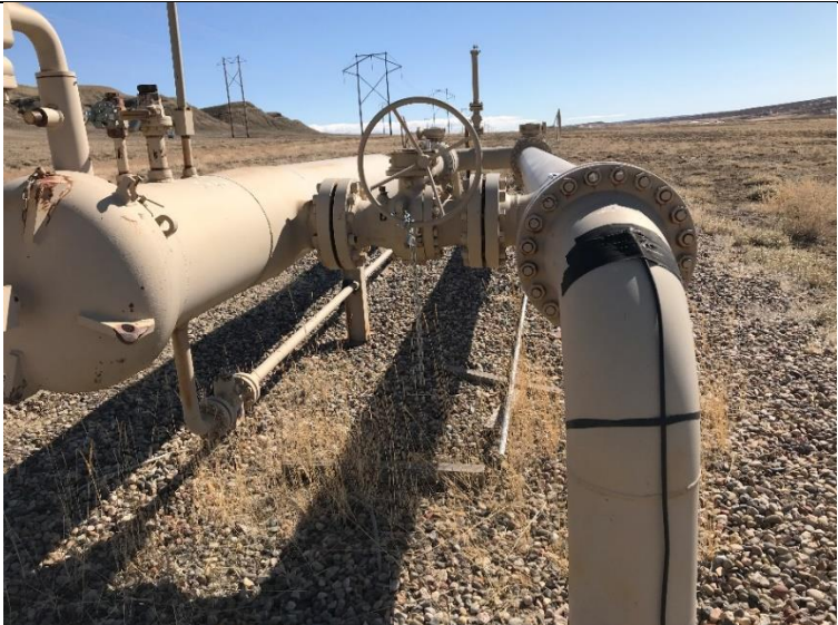
P12. V#6 – Chained and locked in closed position.
