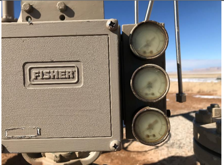
P18. Pressure gauges next to V#10 – indicating zero pressure.
