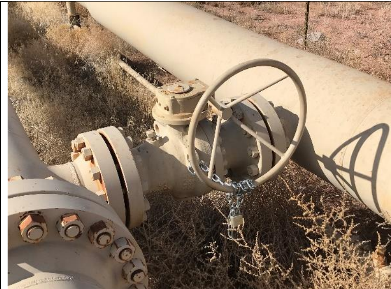
P29. V#19 – Chained and locked in closed position.
