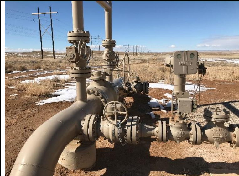
P13. Valve assembly outside Blue Hills Plant.
