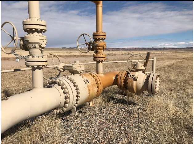
P20. BV#14, and V#s 15, 16 & 17 – Chained and locked in closed position.
