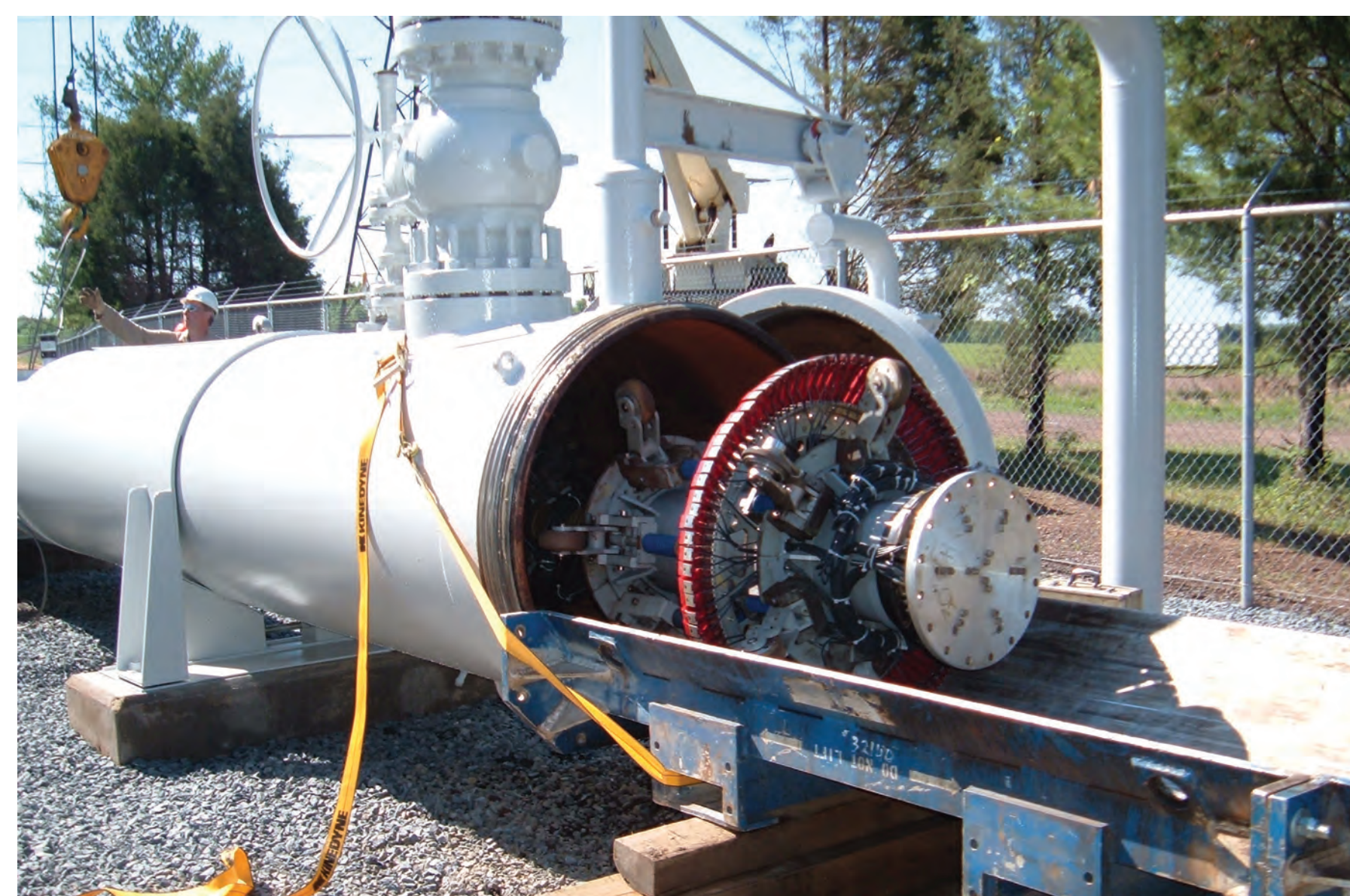
Although pipelines operate underground, in-line inspections can be conducted using smart pigs.
