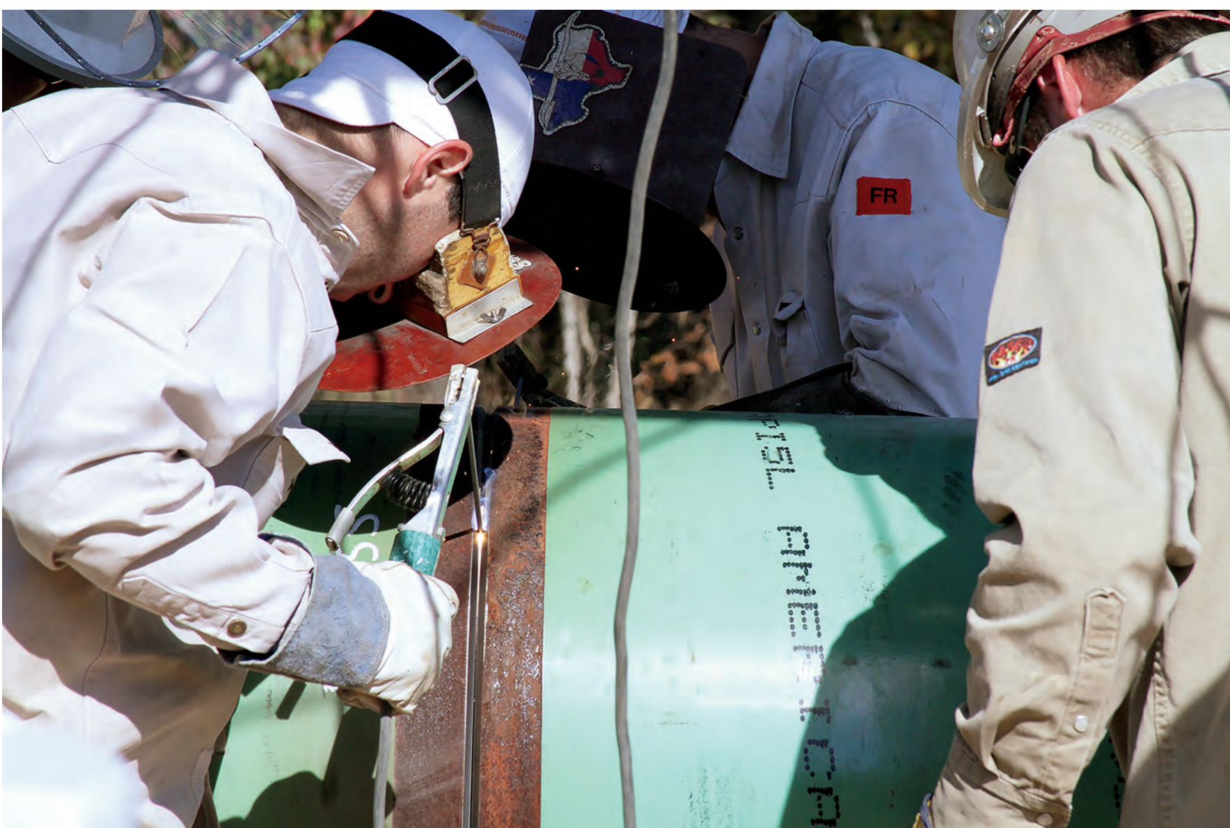
Skilled welders join sections of pipe. Each individual weld is inspected multiple times.
