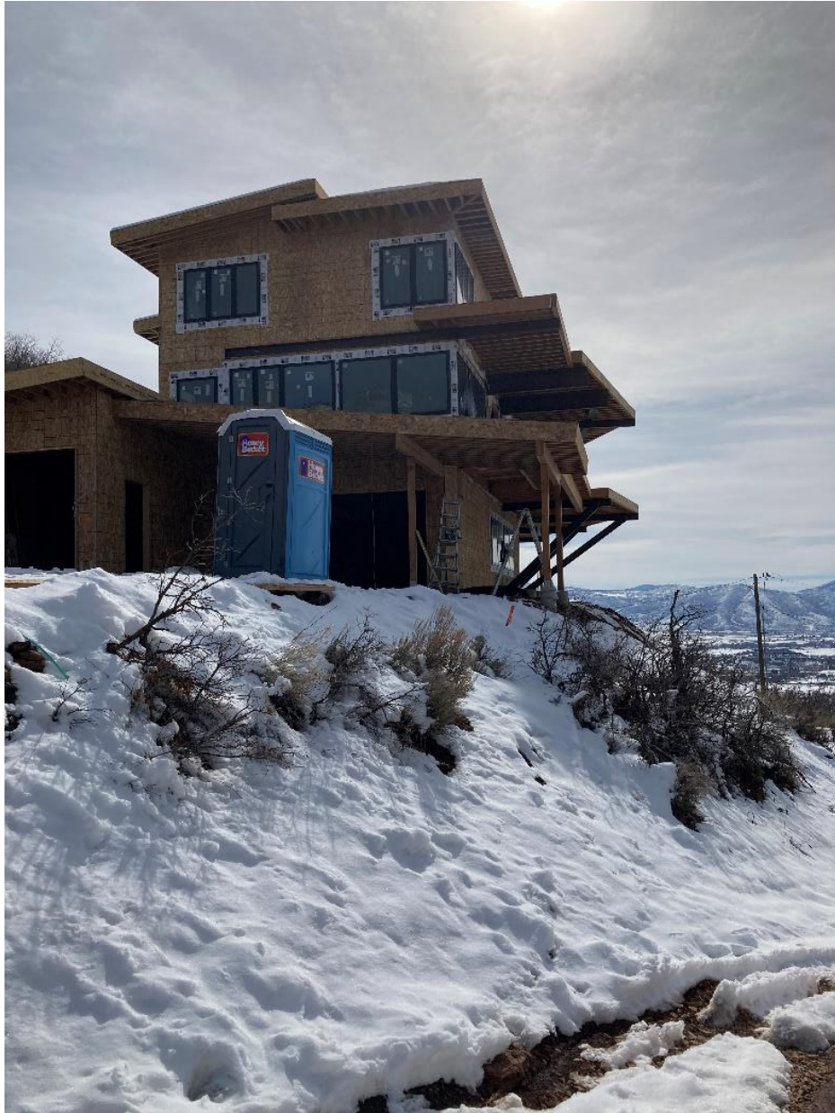
Northside 259, looking South
