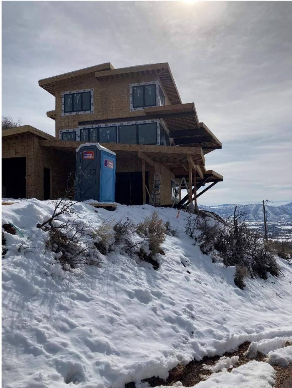
Northside 259, looking South
