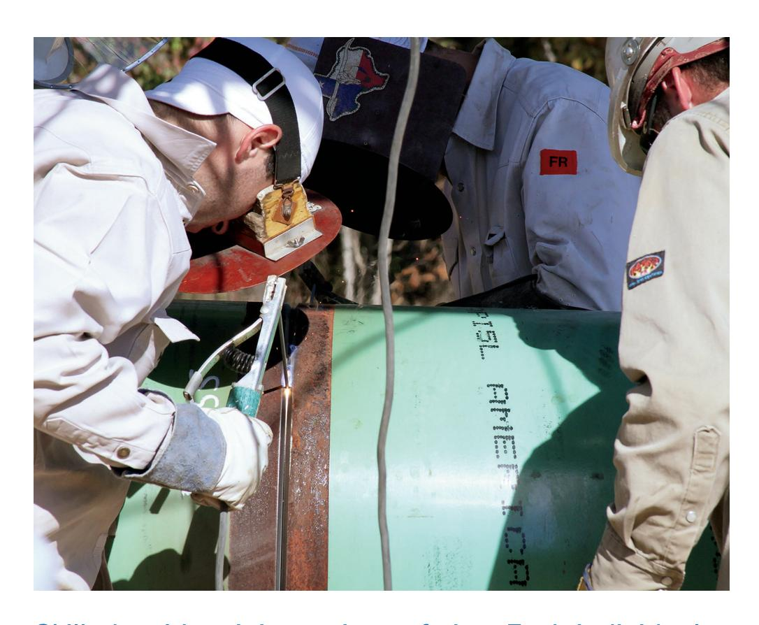
Skilled welders join sections of pipe. Each individual weld is inspected multiple times.
