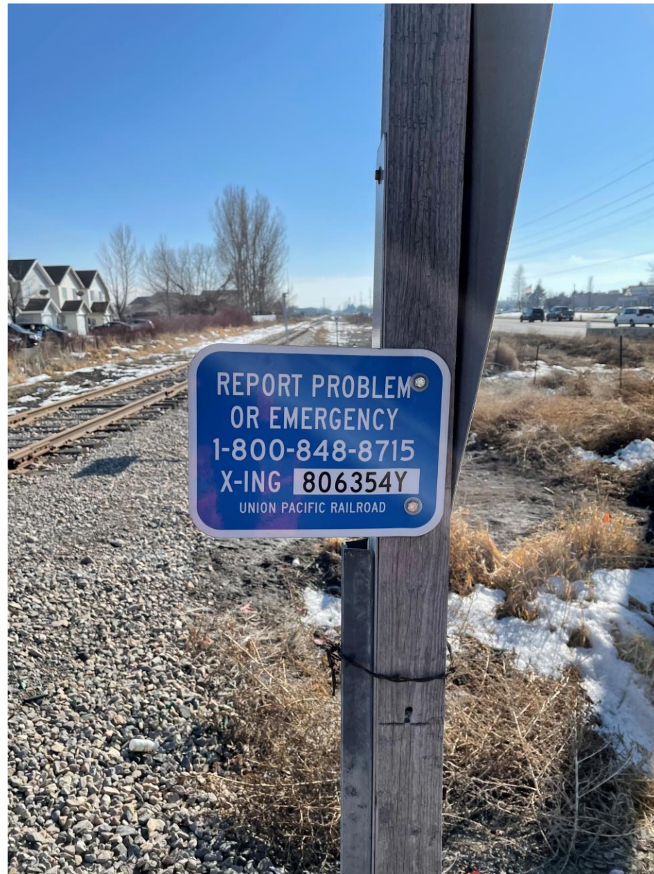
ENS Sign with DOT at Crossing
