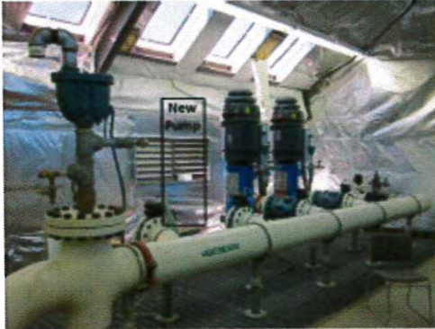
Figure 7: New pump position in the Old Ranch Rd. pump station
