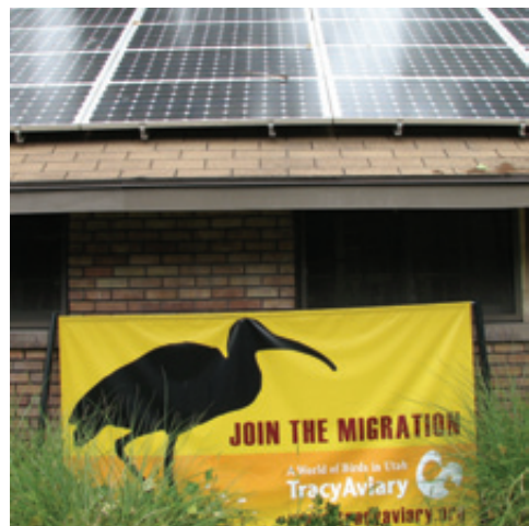
New solar panels will help power Tracy Aviary's Lory Building, while offsetting about 9.5 tons of carbon dioxide emissions each year.
