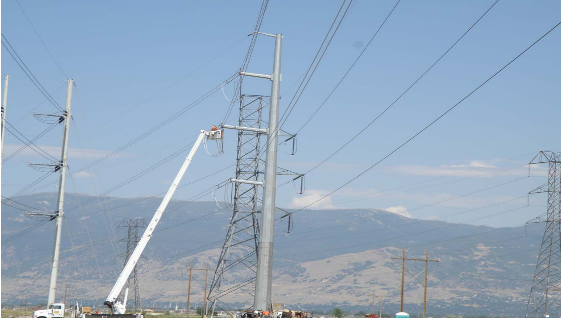
Angle Structure installation Ben Lomond to Terminal
