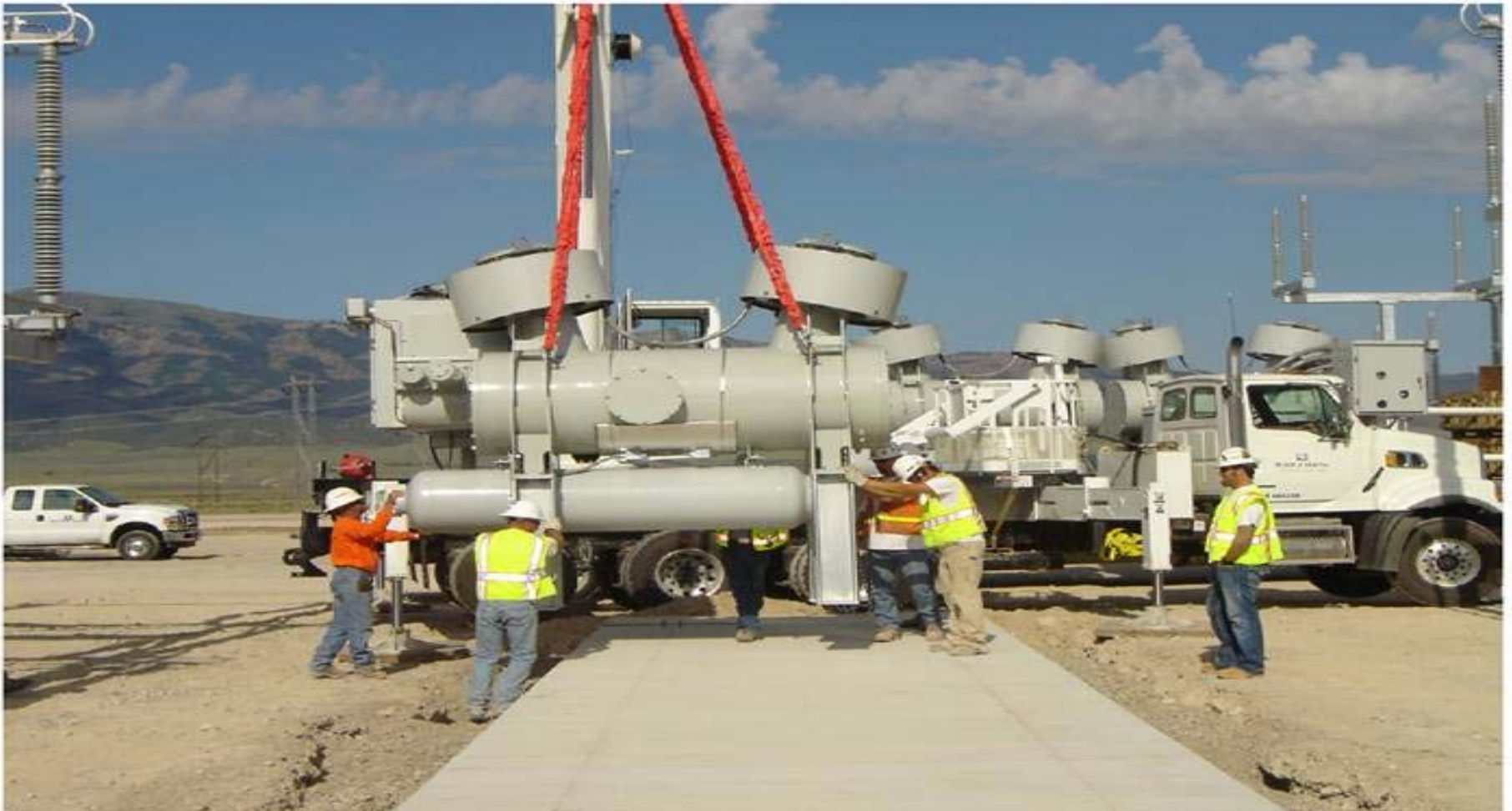
Populus substation (Downey Idaho) – Placing 345kV circuit breaker
