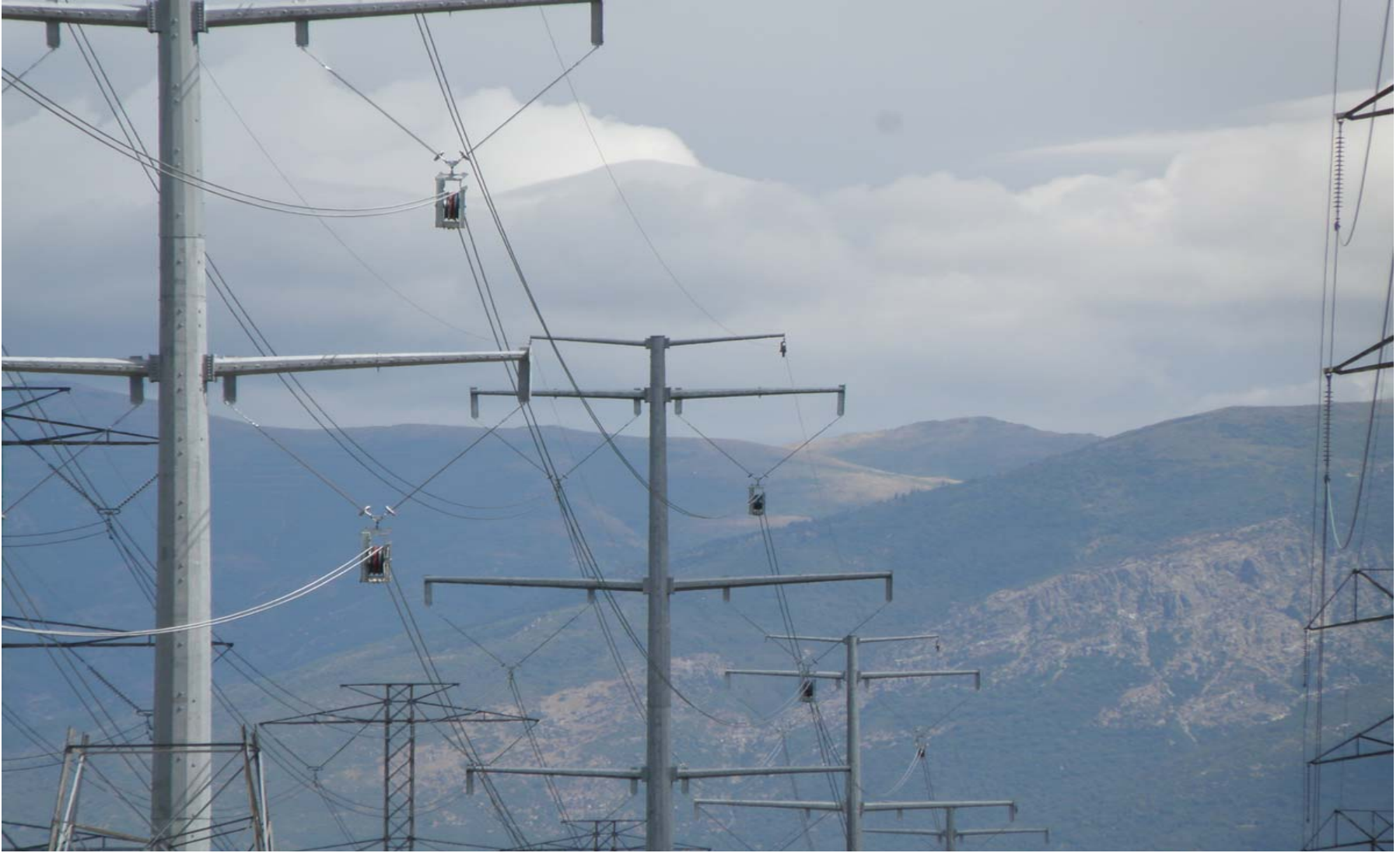
Conductor installation in Ben Lomond to Terminal
