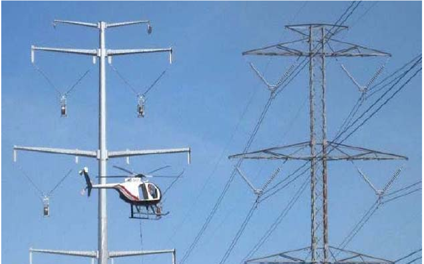
Stringing Optical Ground Wire on Ben Lomond to Terminal
