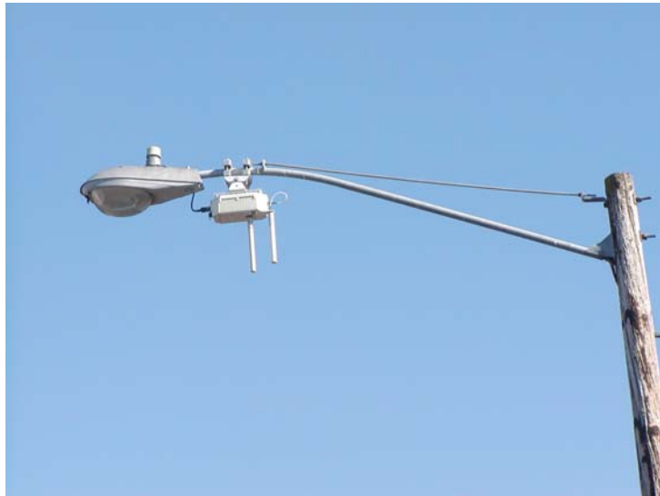
Figure 1—Typical Wi-Fi Antenna Installation on Streetlight Pole
