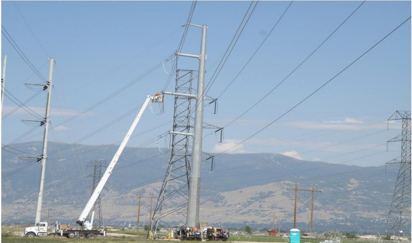
Angle Structure Installation
