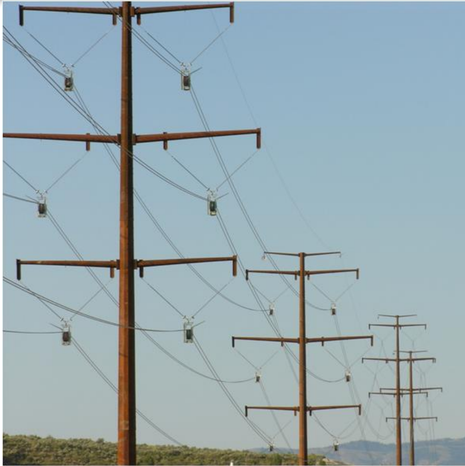
Populus to Ben Lomond section – installed poles
