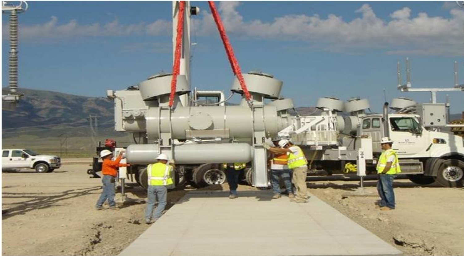
Populus substation– Placing 345kV circuit breaker
