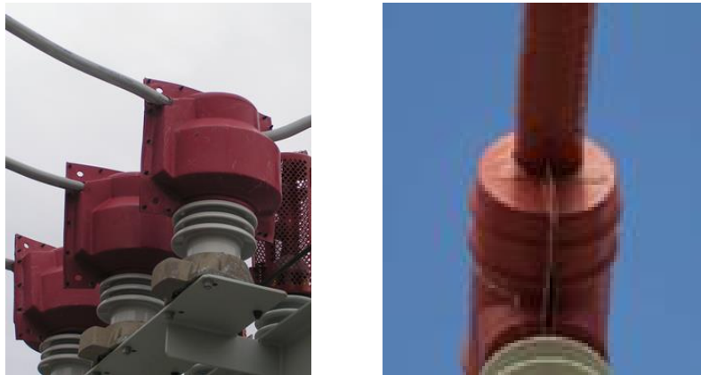
Figure 9—Precise Holes Cut Around Conductors to Prevent Gaps
