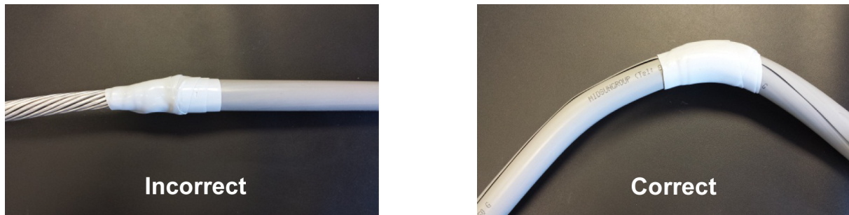
Figure 19—Incorrect and Correct Installation of Self-Adhesive Tape
