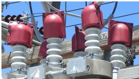
Figure 12—Extra Pins Added to Prevent Gaps Adjacent to Conductors
