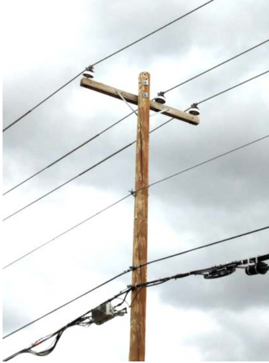
Figure 4—Three-Phase Primary Pole, Example
