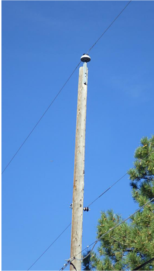
Figure 2—Single-Phase Primary Pole, Example
