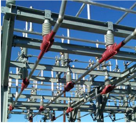
Figure 4—Correct Installation of Heat-Shrink Tape (or Hose) on the Bus
