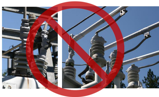
Figure 15—Inappropriate Use of Self-Adhesive Tape
