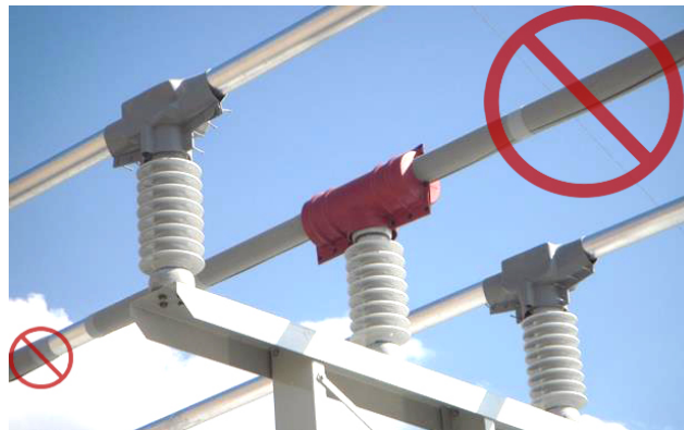
Figure 3—Incorrect Installation of Hose on the Entire Length of the Center Bus
