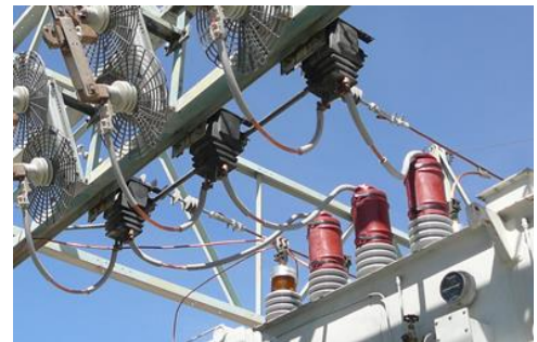
Figure 1—Gaps in Hose Coverage on Conductors for Proper Grounding
