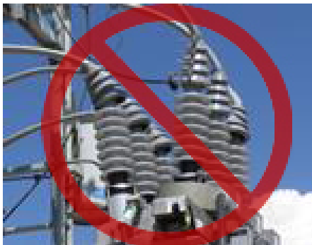
Figure 7—Incorrect Installation of Bushing Covers
