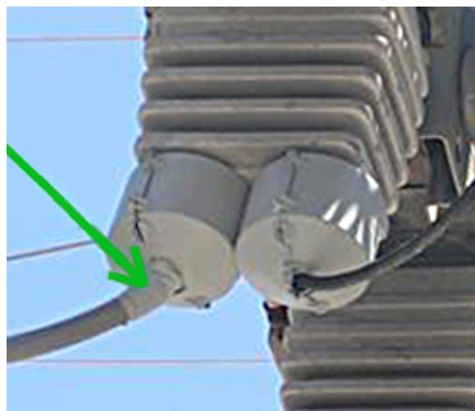
Figure 18—Appropriate Use of Self-Adhesive Tape
