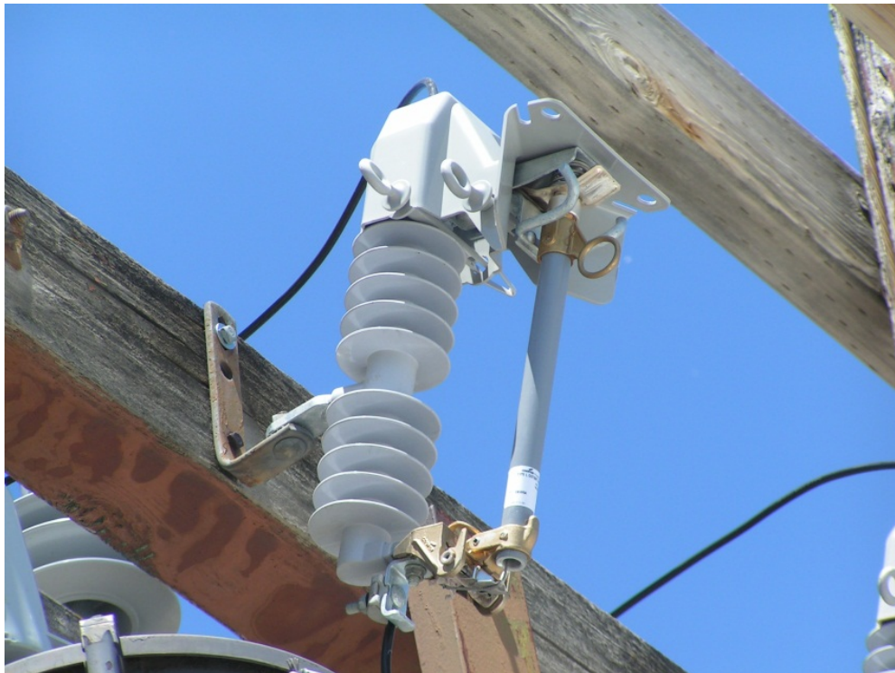
Figure 5—Cutout, With Bird and Animal Protection
