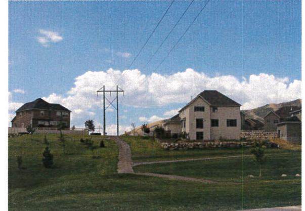
*The area under a transmission line is used to create a path and greenway providing a needed amenity for the community*
