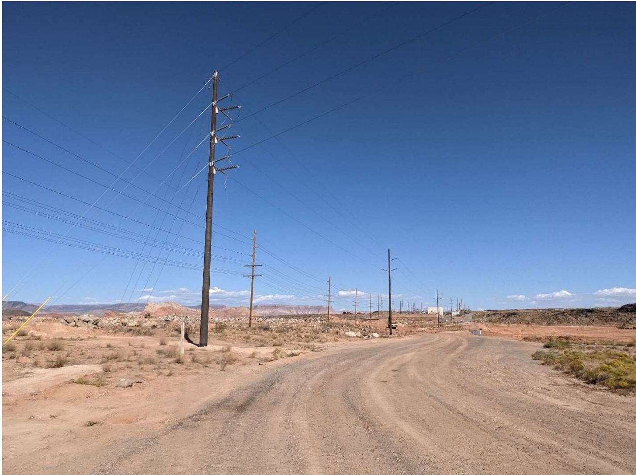
Figure 4: Some of the new steel poles that replaced old wooden poles in 69kV transmission line to the Quail Creek hydro (see in the distance.)
