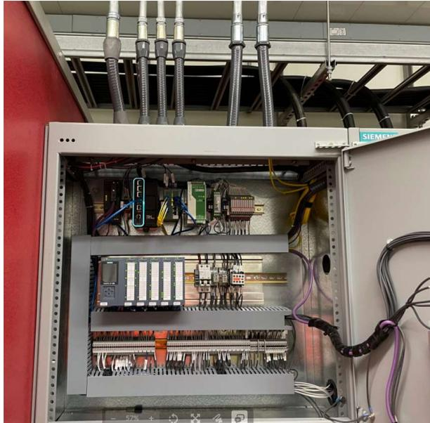
**Figure 36 - Upgraded Red Lion device to TPSS Siemens system. USU connected a cellular device to pull data for algorithm input.**
