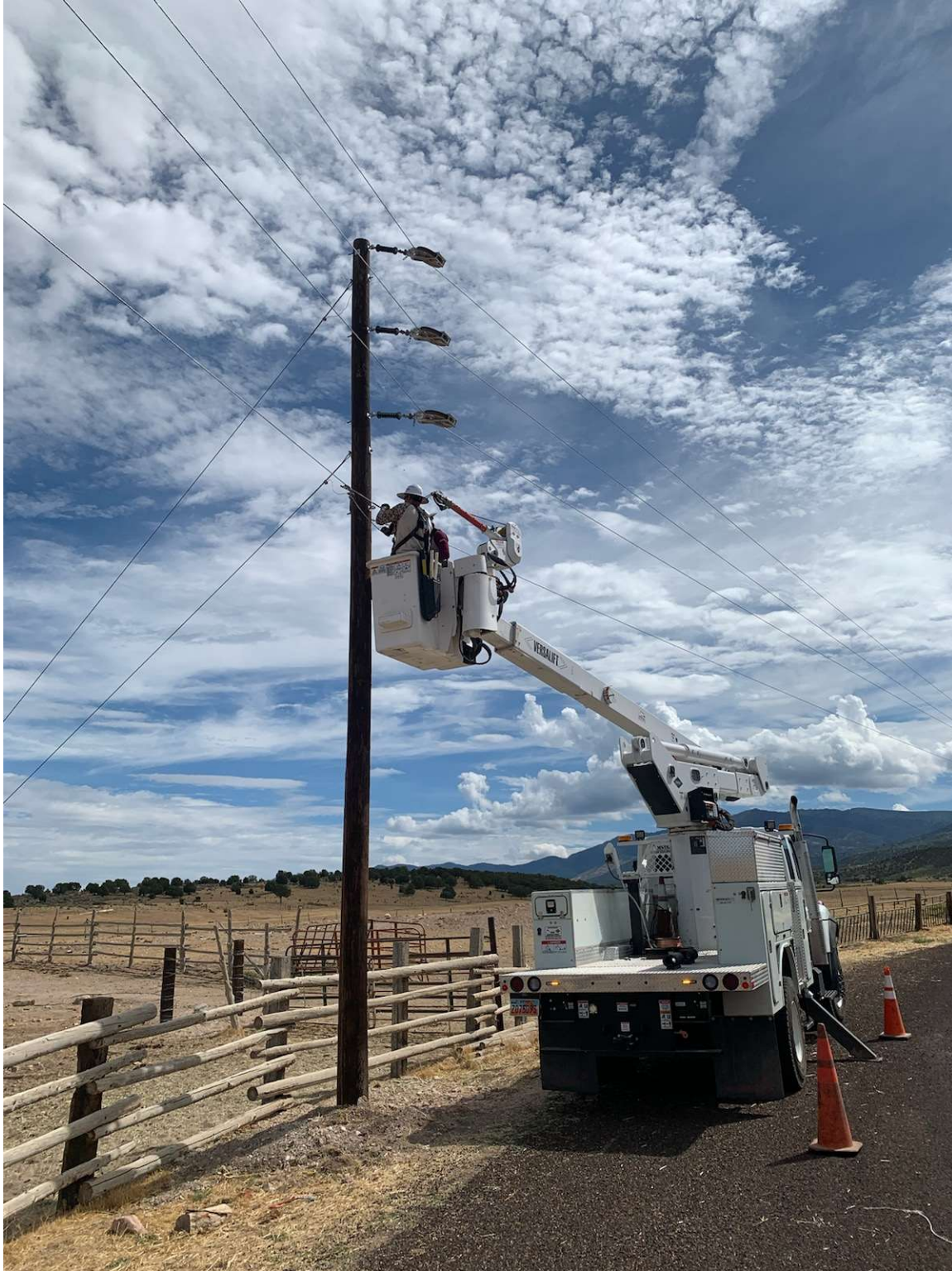
Figure 2: Dixie Power line crews rebuilding the line in segment 411-1.
