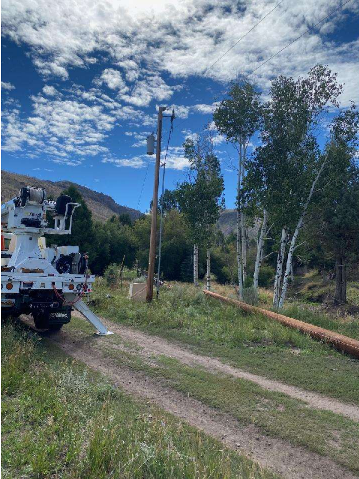
Figure 4: Dixie Power crews working to replace the old powerlines in segment 301-1
