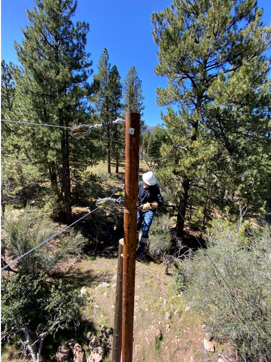
Figure 6: Dixie Power crews working to replace the old powerlines in segment 321-1.
