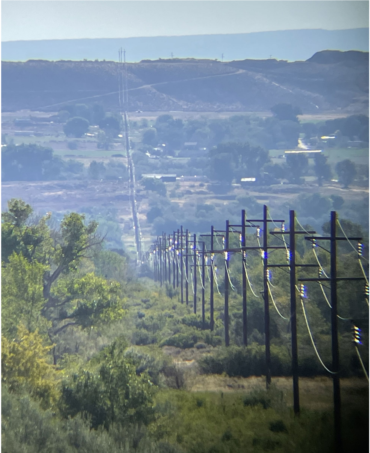
Figure 16. MLEA vegetation management done on a stretch of 69kv line 2022.
