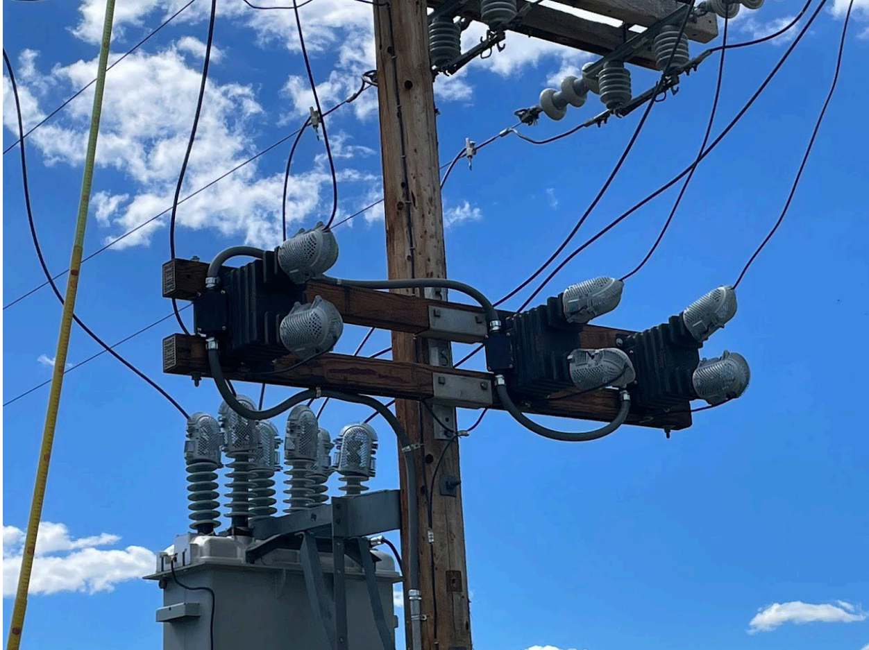
Figure 2. MLEA is installing more reclosers with SCADA control 2023.
