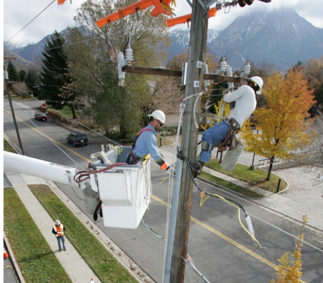
Figure 19: Lineworkers Preparing a Pole for New Covered Conductor
