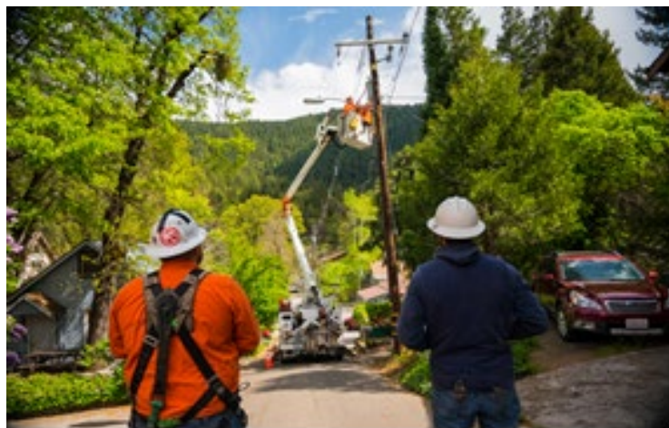
Figure 36: Lineworkers Performing Work
