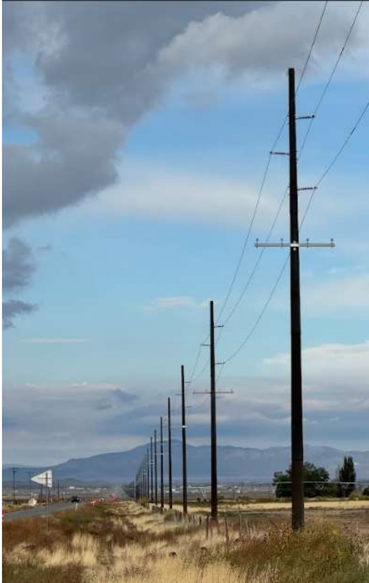
Figure 3: The completed new transmission line with distribution underbuild
