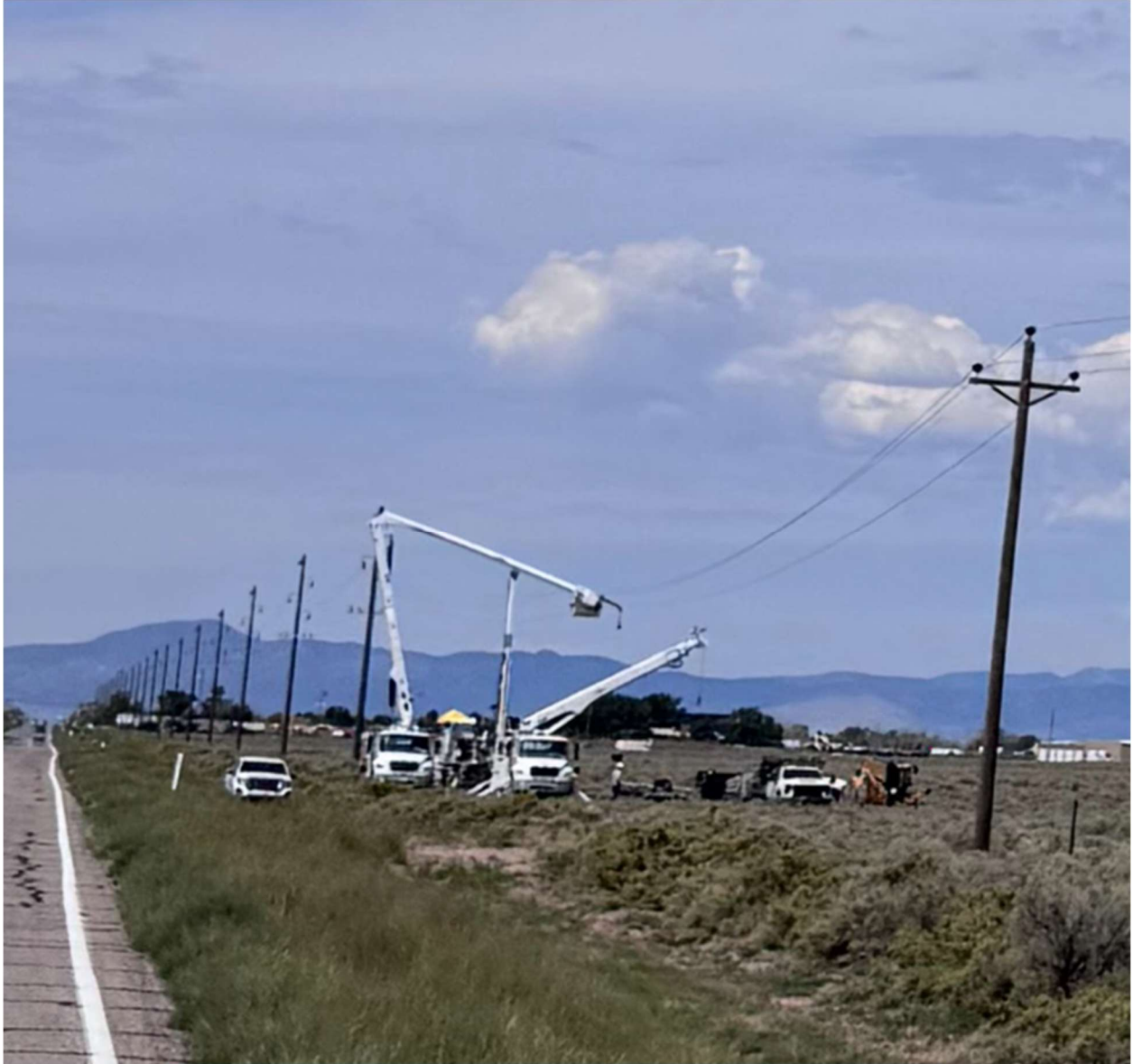
Figure 2: Dixie Power crews working to replace the old powerlines in segment 112-1 & 131-1
