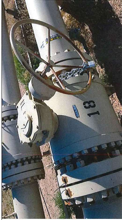
Picture #3: Block Valve BV-18, observed in close position with chain and lock.
