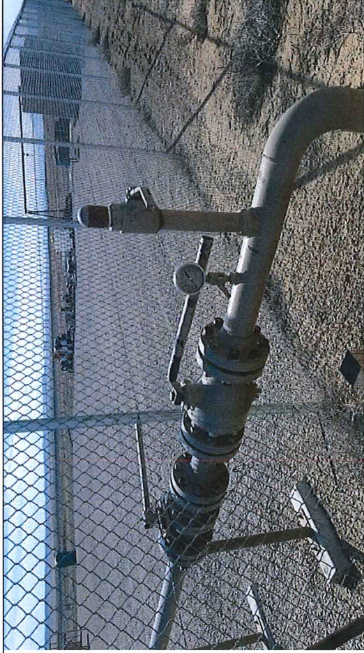
Picture #18: Observe Wesco Compressor Station at Blue Hills, PEMC Valve open position.
