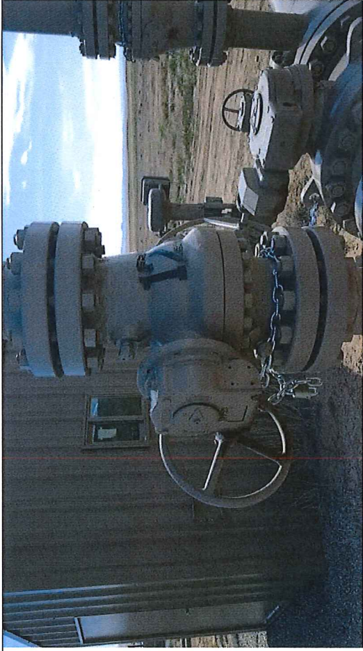
Picture #14: Block Valve BV-12, observed in close position with chain and lock.
