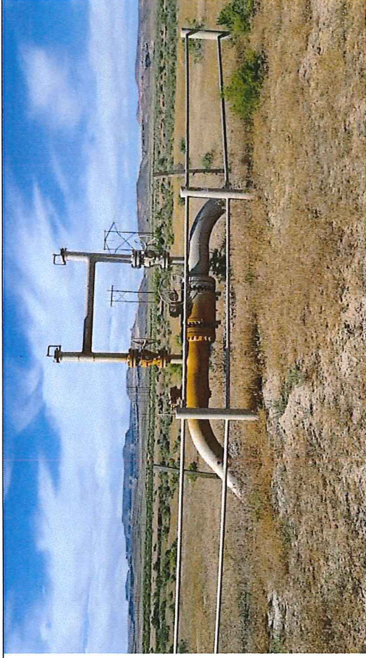
Picture #5: Block Valve assembly BV-14, BV-15, BV-16, and BV-17.
