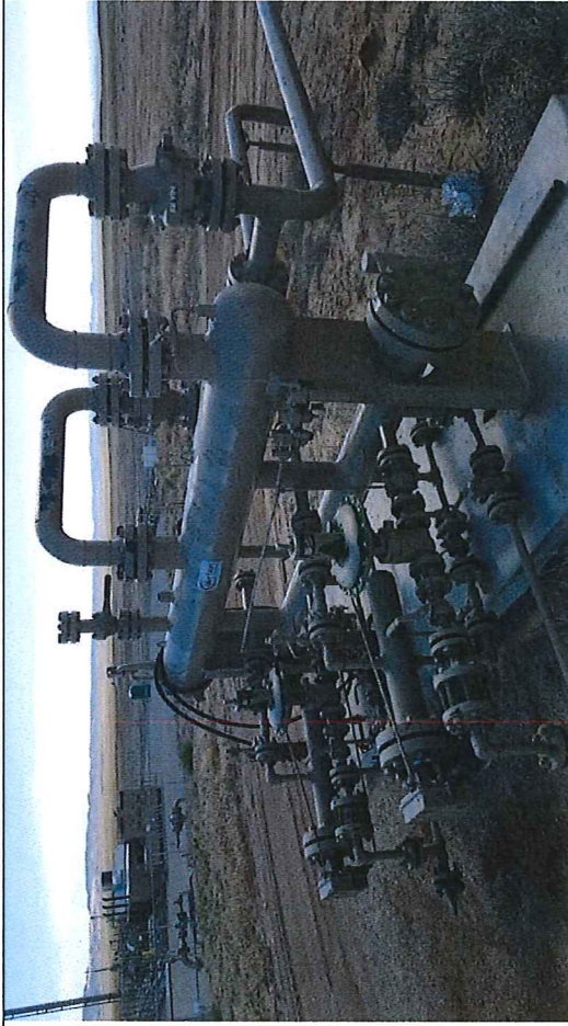
Picture #14: Block Valve BV-12, observed in close position with chain and lock.
