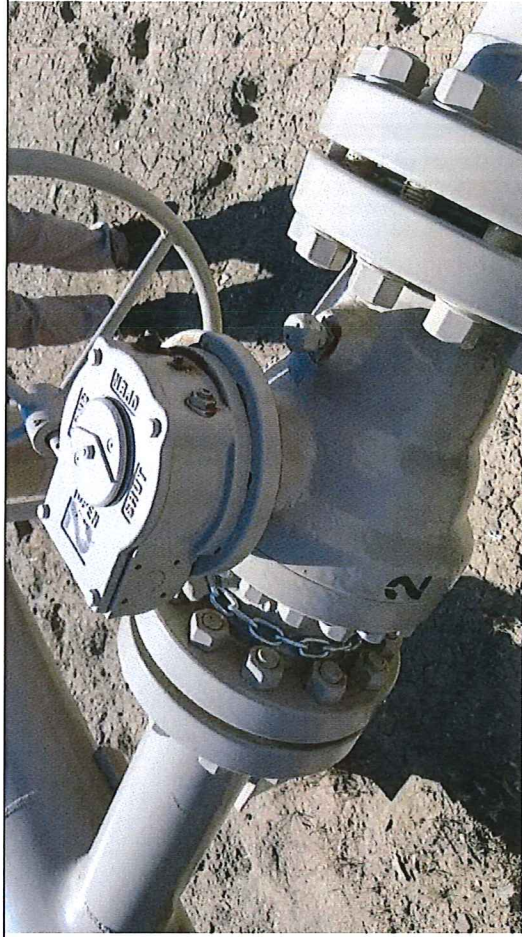
Picture #32: Block Valve BV-2, observed in close position with chain and lock.
