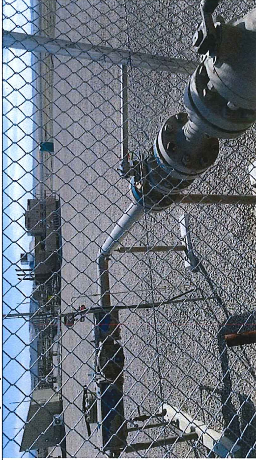
Picture #18: Observe Wesco Compressor Station at Blue Hills, PEMC Valve open position.
