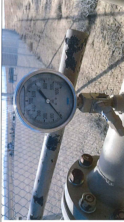
Picture #19: Observed Wesco Compressor Station at Blue Hills pressure gauge approximately 0 psig.
