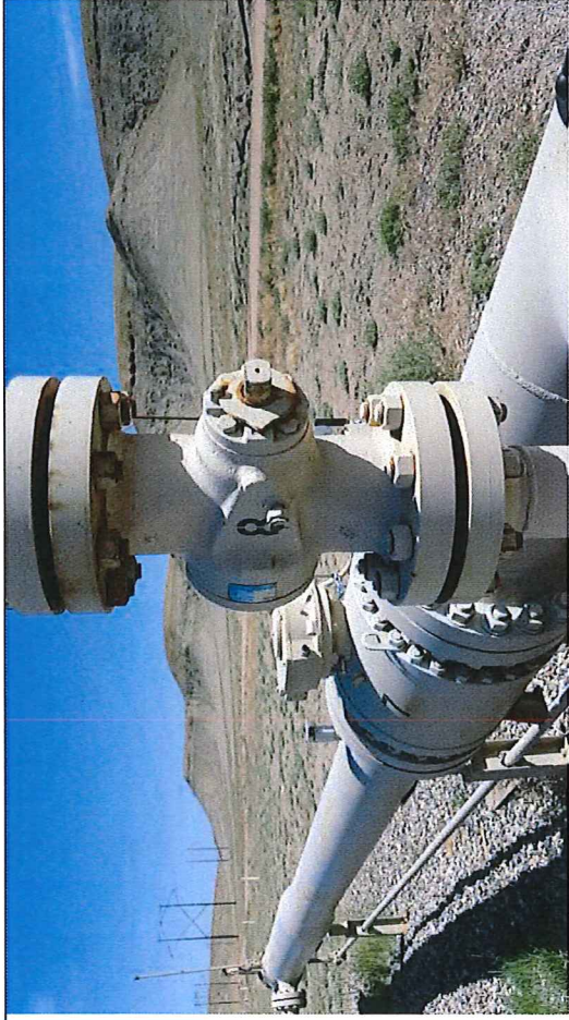
Picture #25: Block Valve BV-8, observed in close position with chain and lock.
