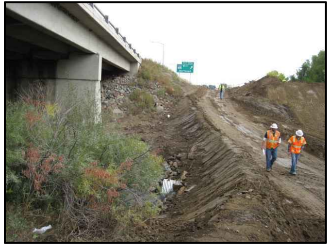
Temporary Berm along access road
